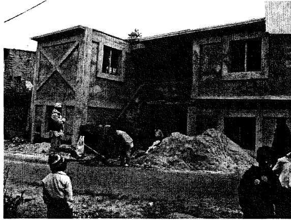
Figure 11: A Retrofitted School Building
