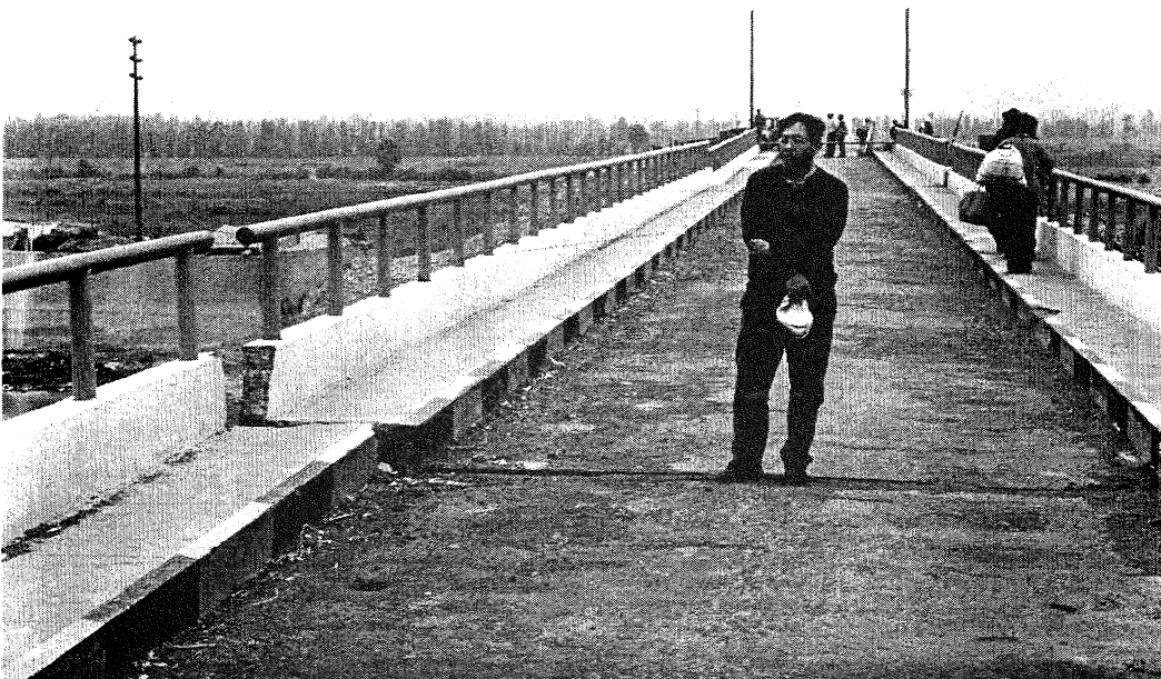
Figure 12. Damage to the bridge serving the township of Punta De Bom Bon.
