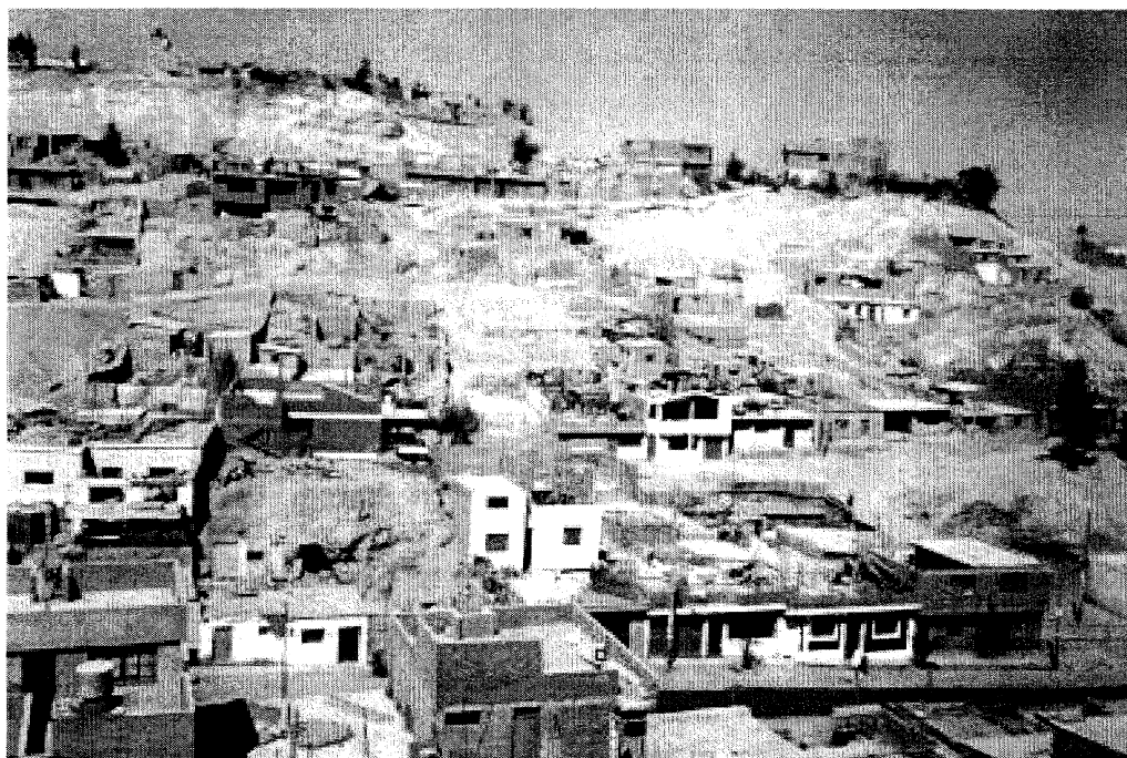
Figure 9. Severe damage to buildings on the steep hillslopes of Moquegua. These hillslopes, along with the valley bottoms, are underlain by alluvial sediments which would have amplified the shaking from the earthquake. In this photograph nearly all adobe buildings have been destroyed, with considerably less damage to the more substantially constructed buildings.
