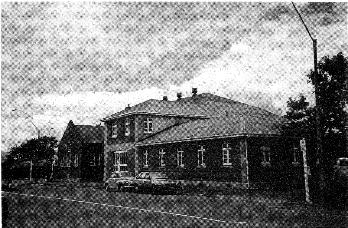
Figure 9: Present day views of 2-storey 1938 Knox Church Hall in Masterton, with a reinforced concrete frame and brick infill, which suffered little or no damage during the 1942 earthquakes. (Photograph by D.J. Dowrick, 1998).
