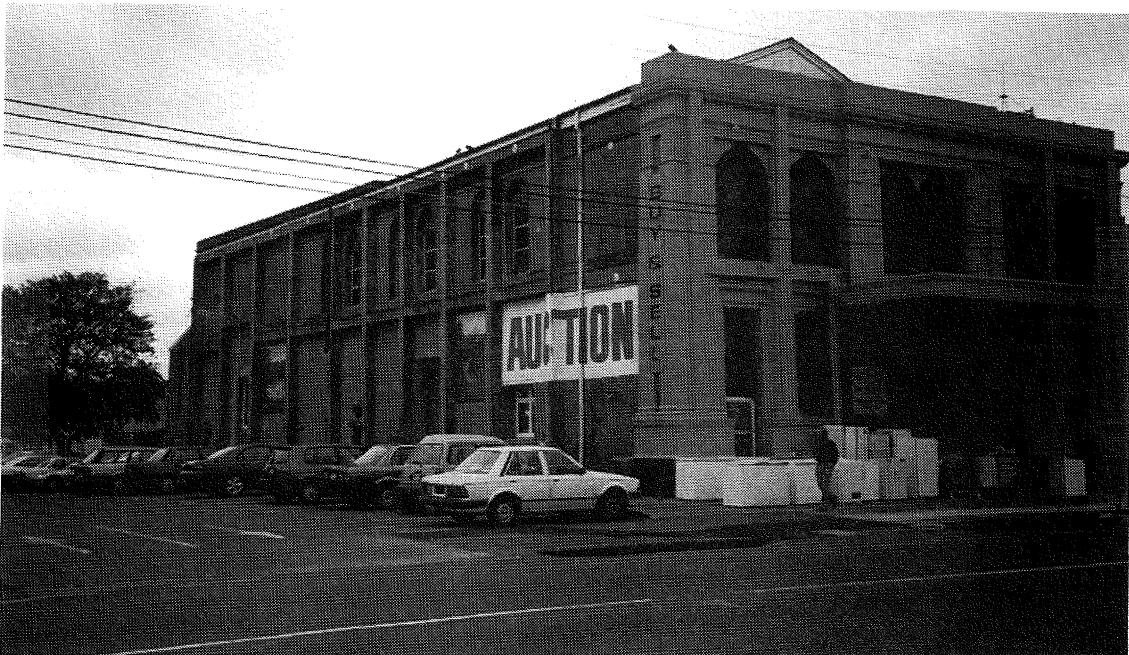
Figure 7: Present day view of the former Opera House, Masterton, showing reinforced concrete beams and columns attached to brickwalls in retrofitting mostly after 1934. (Photograph by D.J. Dowrick, 1998).
