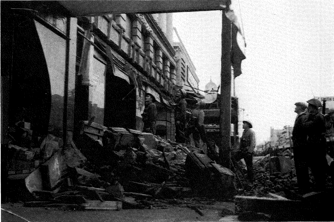
Figure 6: A view of Queen Street, Masterton on June 25 1942. The debris is from the second storey of Gray's brick building housing Hannah & Co., and Bullick & Blackmore. The undamaged parapet of Woolworth's single storey 1937 reinforced concrete building may be seen just beyond Gray's. (Reference No. G-123912-1/2, "Evening Post" Collection, Alexander Turnbull Library, Wellington, New Zealand).
