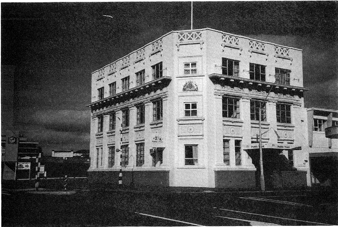
Figure 8: Present day views of 3-storey 1922 wholly reinforced concrete Public Trust building in Masterton, which “suffered no structural damage whatsoever” during the 1942 earthquakes (PGA=0.3-0.6g). (Photograph by D.J. Dowrick, 1998).
