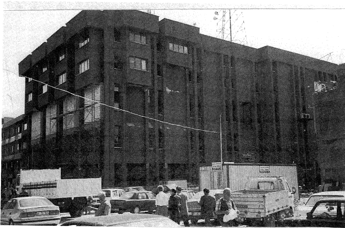
Figure 25: Turk Telekom Building, Adapazari.
