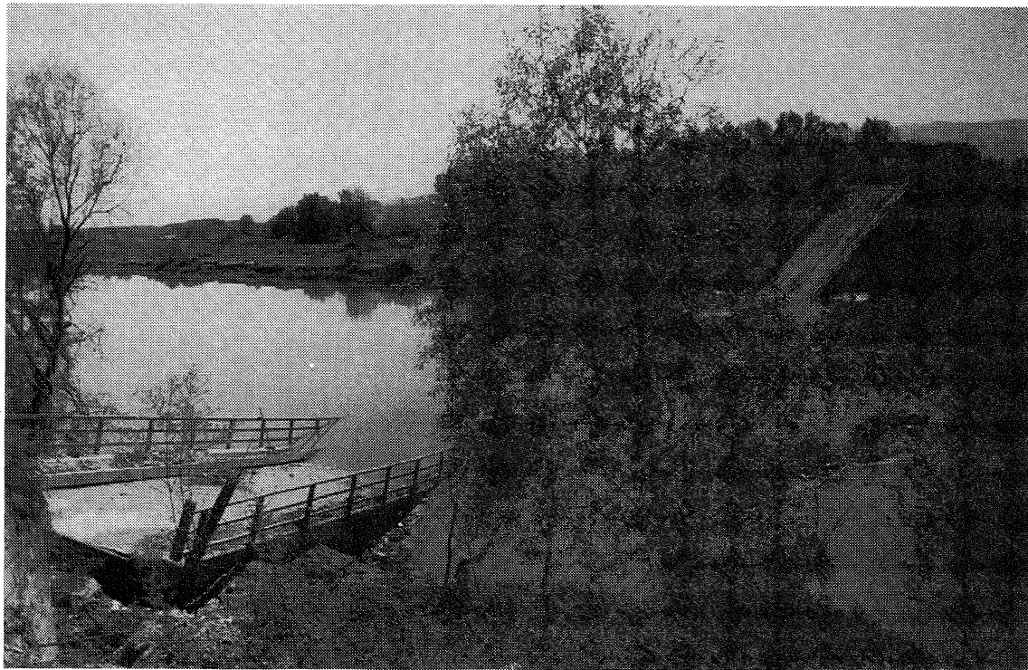
Figure 32: Sakarya River Bridge.
