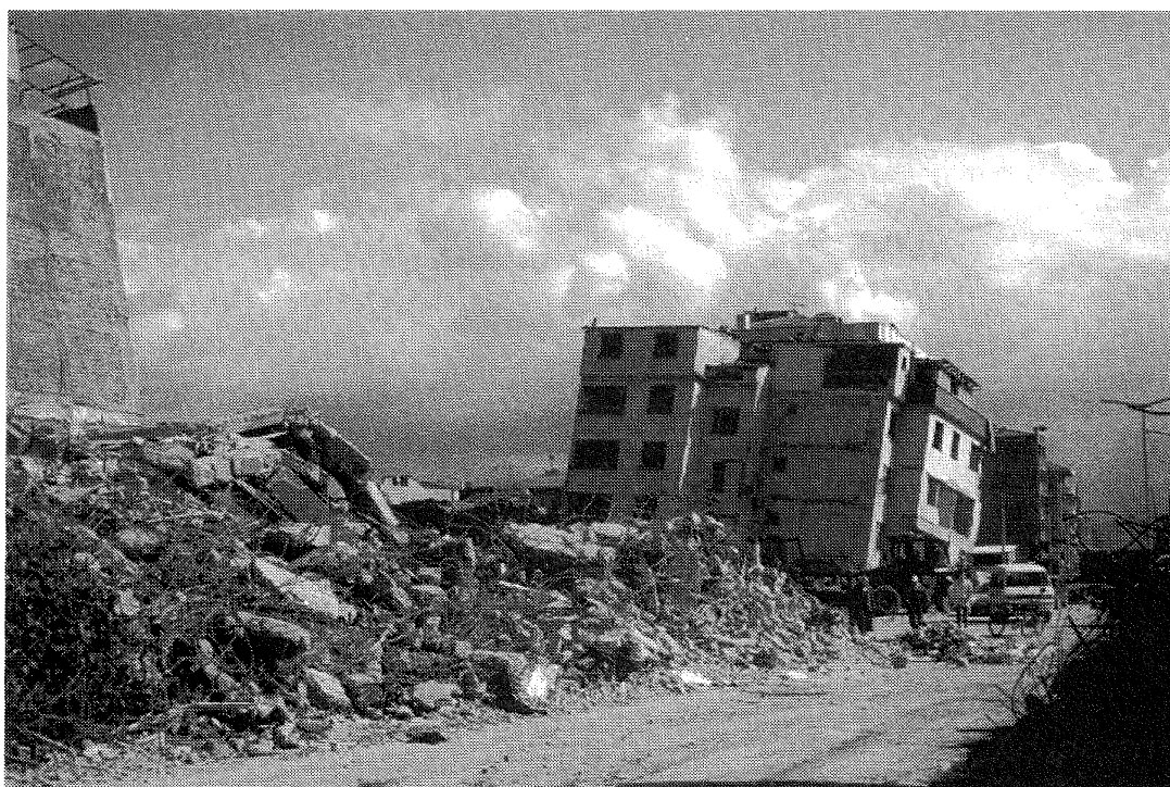
Figure 3: Typical street scene showing devastation of Adapazari.
