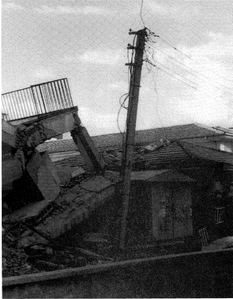
Figure 36: Power pole damaged by collapsing adjacent building.
