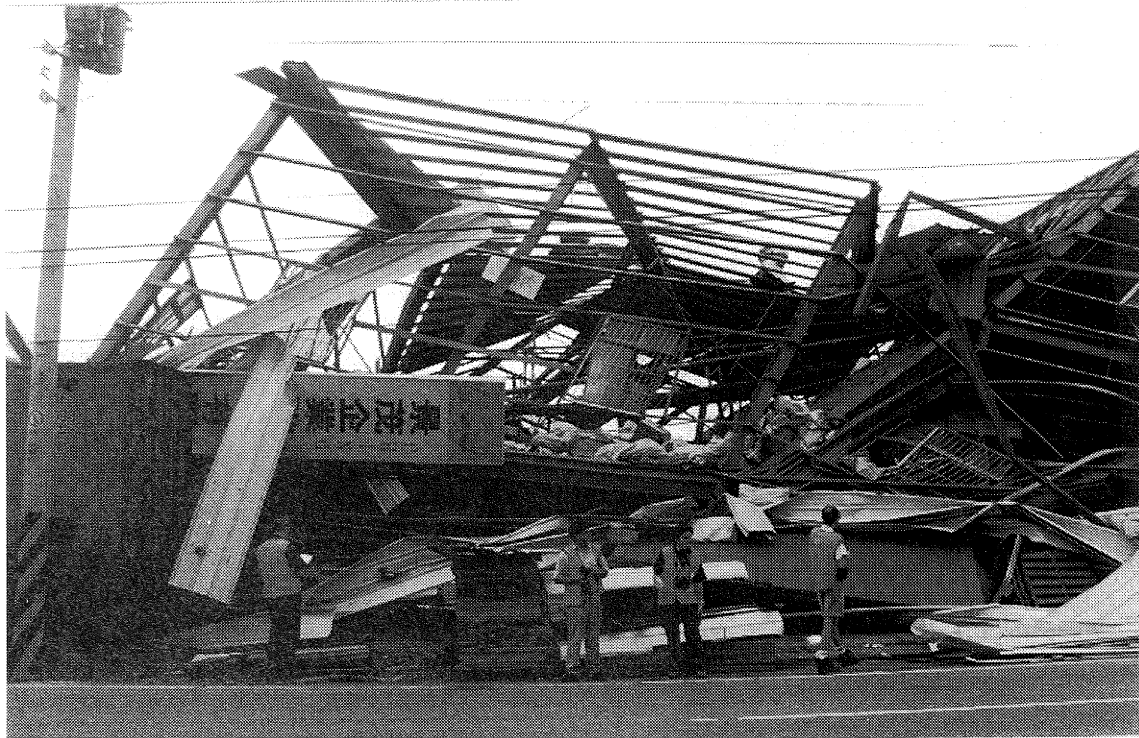
Figure 5.20: Collapse of steel framed building attributable to absence of any bracing or framing in the longitudinal direction.
