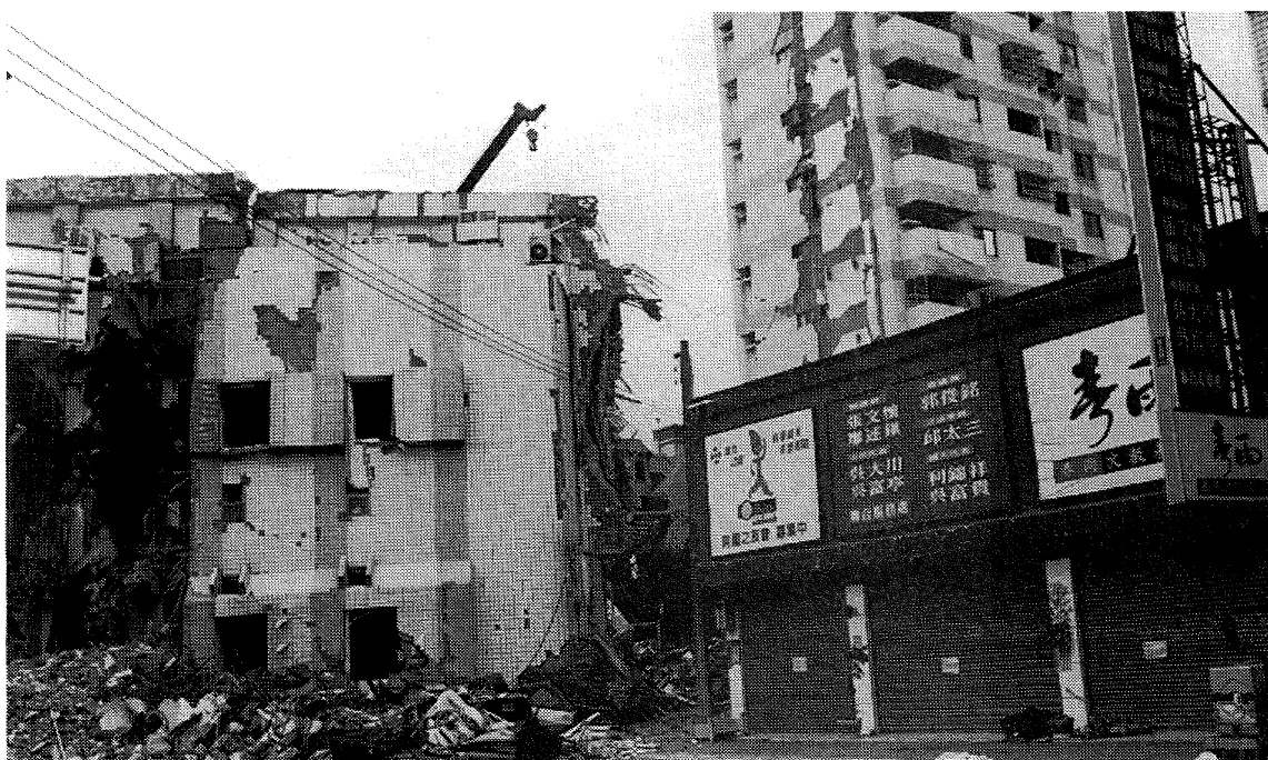
Figure 5.9: Soft storey collapse resulting in toppled building, Fengyuan.
