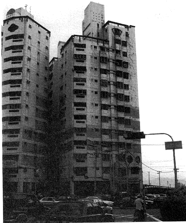
Figure 5.11: Overall view of damaged multistoreyed apartment building, Taichung.
