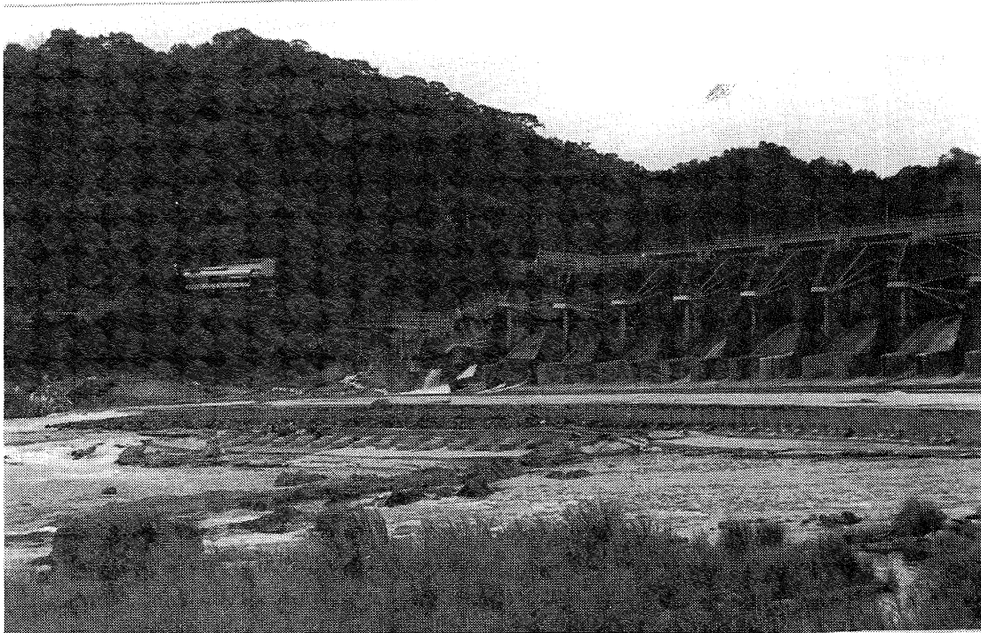
Figure 7.1: Damage to Shih-kang Dam.
