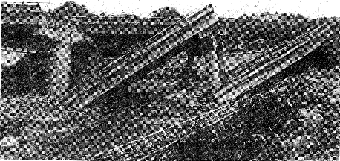
Figure 6.1: Collapsed spans of prestressed concrete I beam bridge crossing the Tachia Hsi river.
