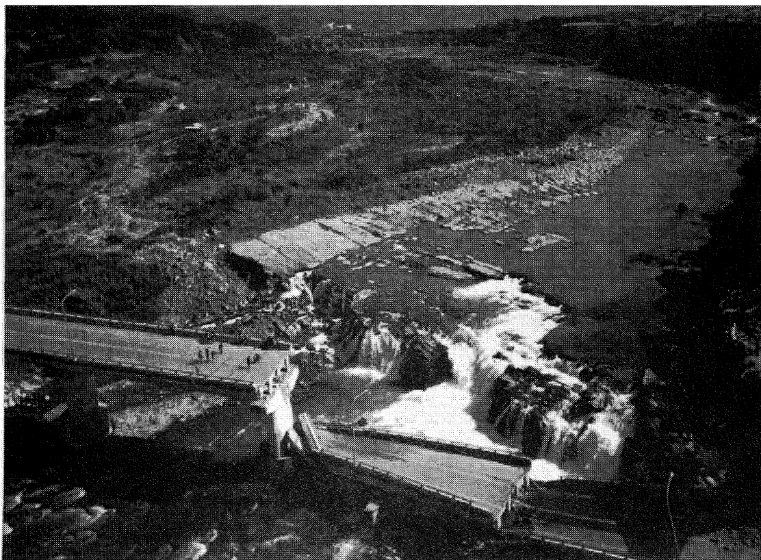
Figure 3.21: Fault rupture passes through the bridge and dam (background) near Shihkang.
