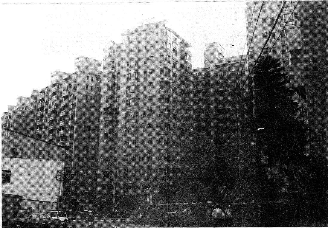
Figure 5.16: Apartment complex in Taichung. Basement carparking and ground floor apartments allow structural form to carry to ground level without significant stiffness variation. Non-structural panels present on all levels.
