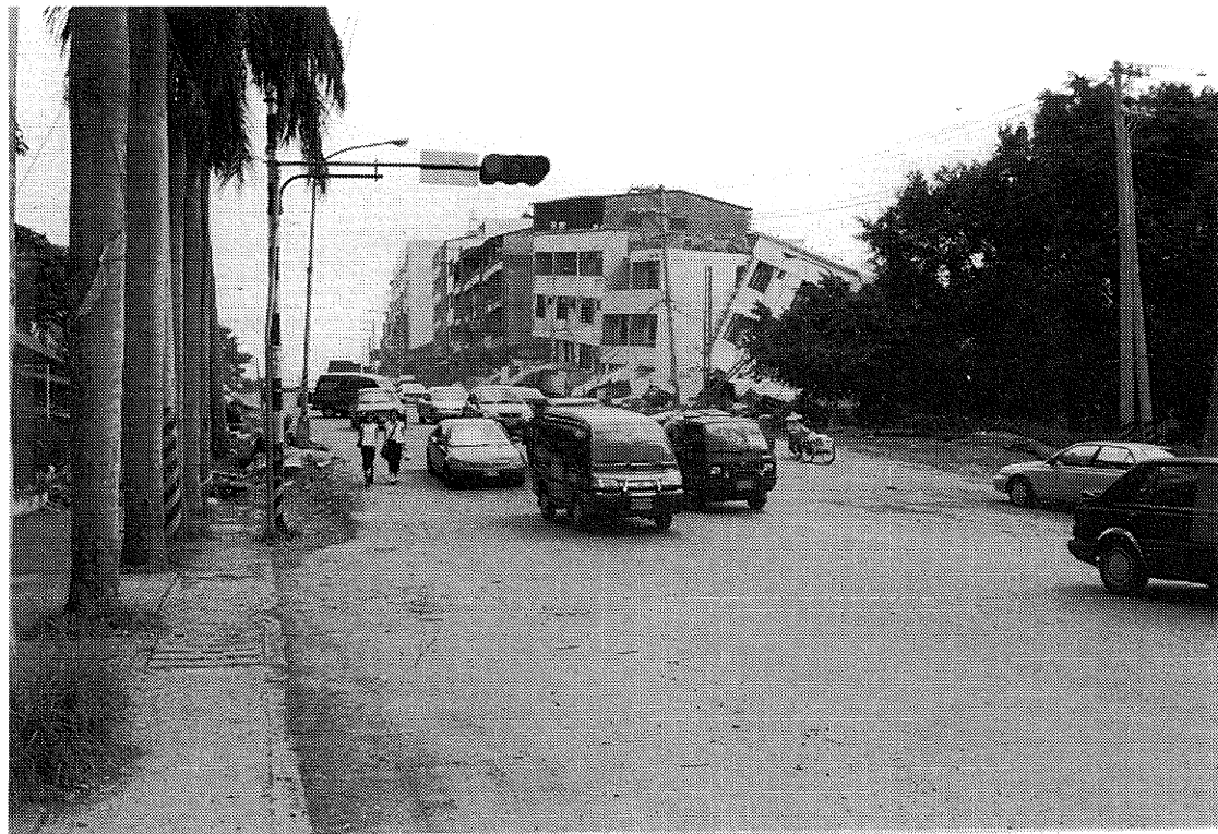
Figure 3.19: The fault scarp near Tsaotun. The scarp deformation shows clearly in the road and in the building damage.
