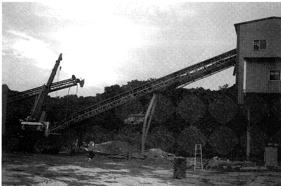
Figure 7.3: Damaged conveyors at concrete plant near Mingchien.
