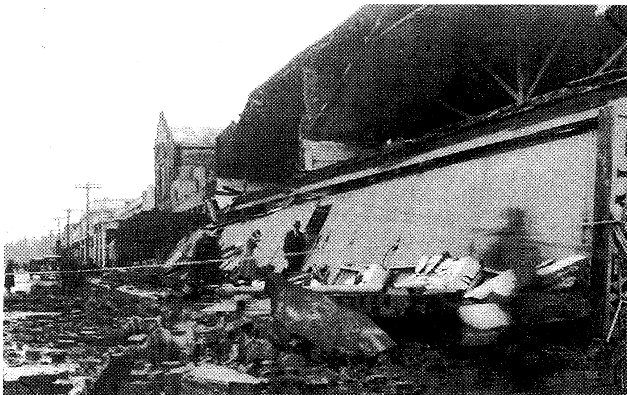
Figure 4. View along the main street of Pahiatua, showing the collapse of the brick facade of the upper storey of the Wairarapa Farmer's Cooperative Association store. (Reference no. P-A1 0832-021 -0, Alexander Turnbull Library, Wellington, New Zealand)
