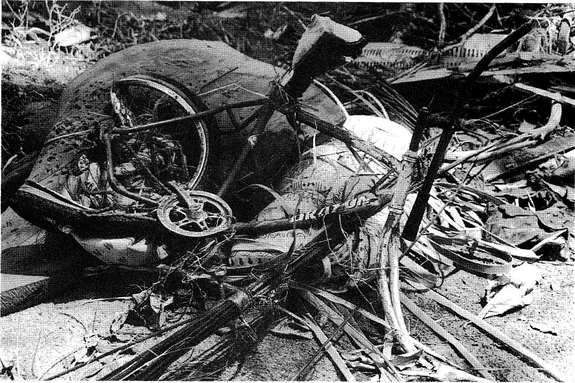
Figure 20: Every major part of this child's bicycle was deformed as it was tossed around in the tsunami.
