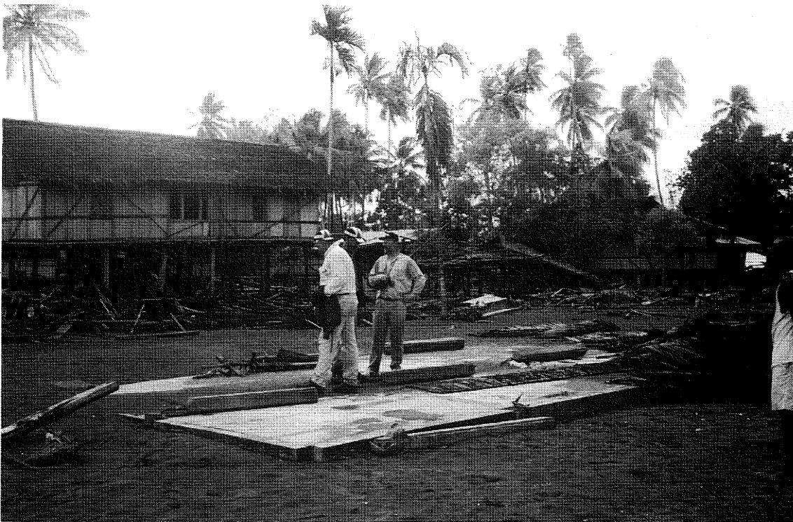
Figure 15: Three members of the reconnaissance team inspect damage at Malol Village. Here tsunami damage was only intermittent along the coast, where ocean swells boosted the tsunami over the beach berm.
