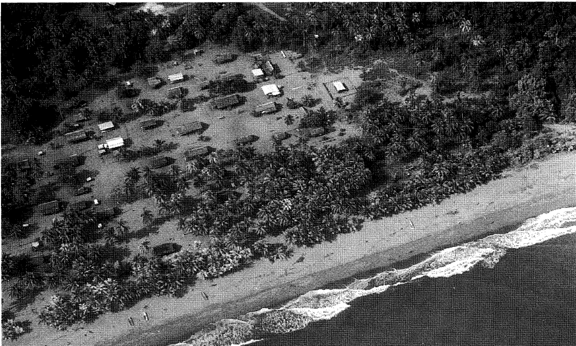
Figure 14: A typical village along the northern coast of Papua New Guinea outside the region of significant tsunami damage. The destroyed villages of Arop and Warapu probably had similar proportions of traditional and iron clad dwellings.
