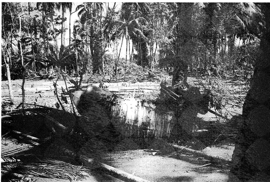
Figure 19: A heavy steel pontoon 1.5 metres in diameter was wrapped around a coconut palm.
