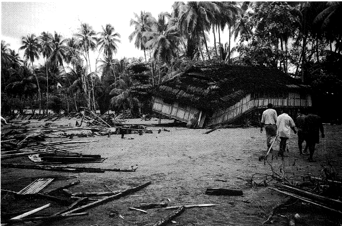
Figure 16: On the lateral edge of a local damaged zone in Malol Village, this traditional style dwelling might have survived intact on more adequate piling. Clusters of tilted piles (left centre and background) indicate sites of destroyed dwellings.
