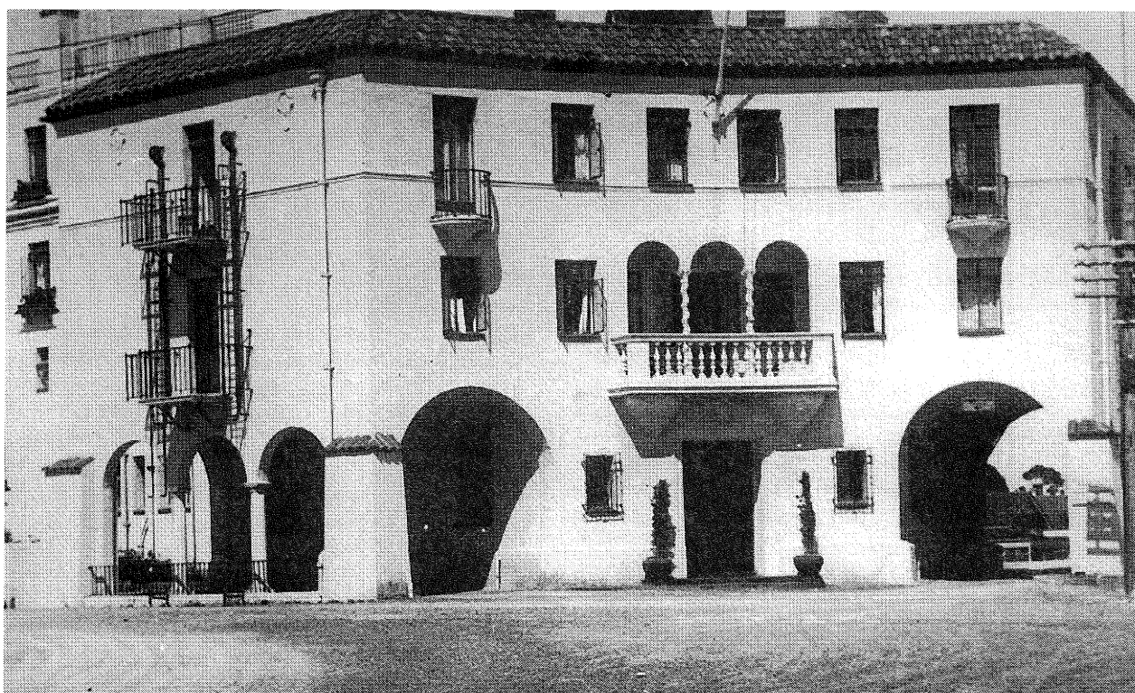
Figure 11: (b) A poor reinforced concrete building. The Nurses' Home at Napier Hospital before the earthquake, the only r.c. building to collapse completely, due to a bottom storey weakened by large openings and little reinforcement (Courtesy of the Alexander Turnbull Library, Wellington).
