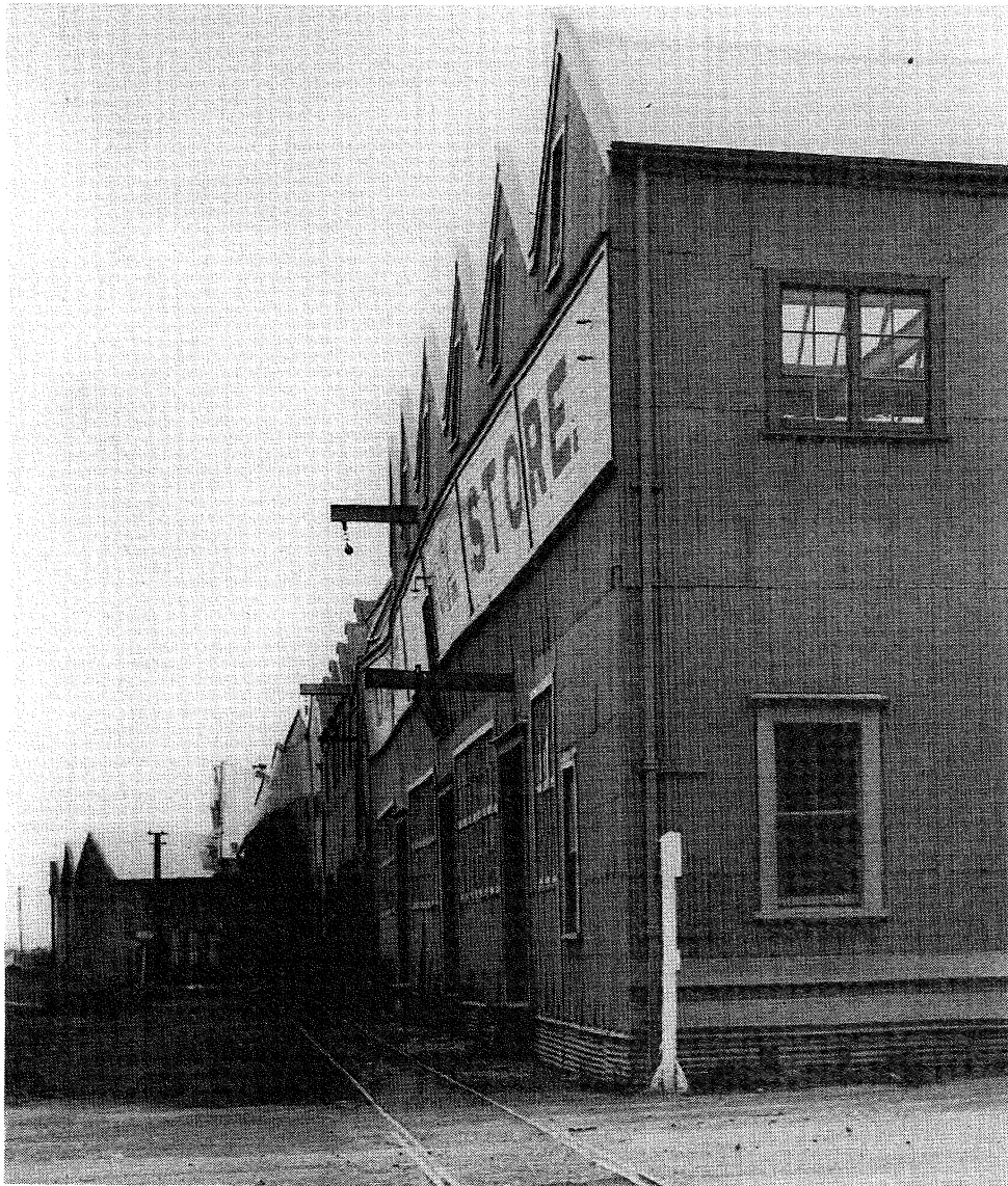
Figure 10: Dalgety's No. 2 Store, Port Ahuriri, Napier one of the few steel-framed buildings in the region, was inadequately braced. (Courtesy of the Alexander Turnbull Library, Insurance Council of NZ Collection, Wellington).
