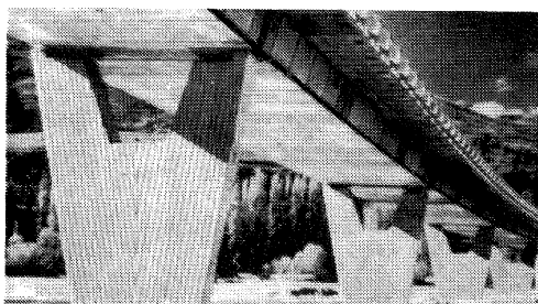
FIGURE 1 Lower Shotover Bridge Constructed Near Queenstown in the 1970s.
