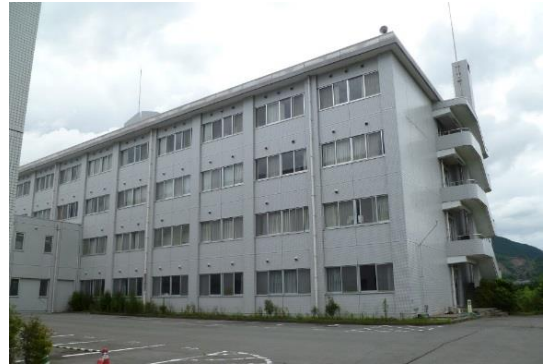
Photo 17: Building A14. Exterior covered in ceramic tiles applied directly to the concrete structure. A typical Japanese cladding system
