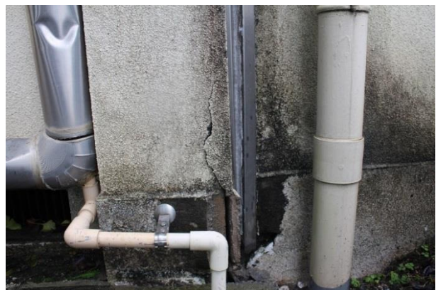
Photo 9: Pounding damage at seismic joint between classroom blocks.
