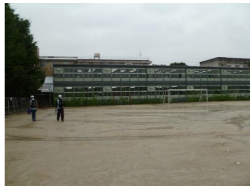
Photo 38: Building A11,, Temporary class room block erected in school playing field
