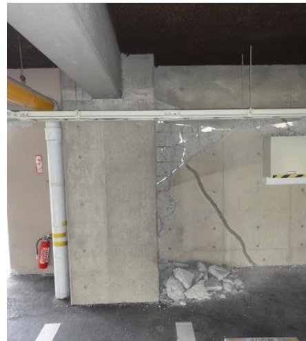
Photo 14: Column adjacent to the north entrance.
