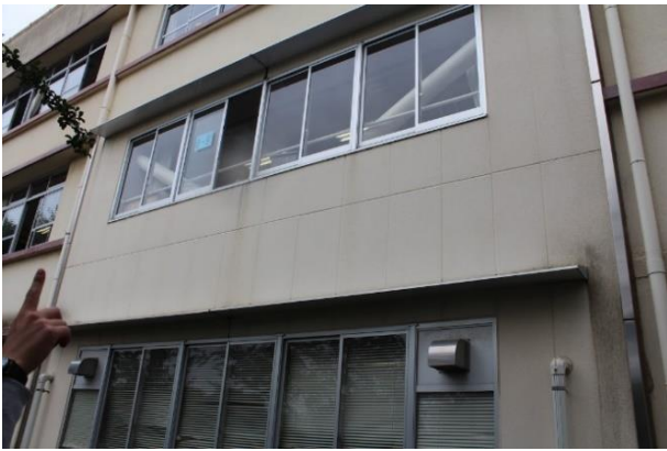
Photo 3: School elevation from playground side.
