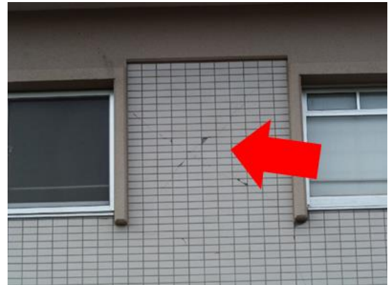
Photo 18: Building A12, Exterior tiled cladding.
