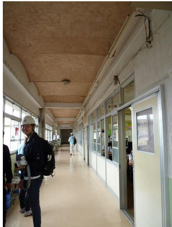
Photo 10: Building A10 classroom corridor.
