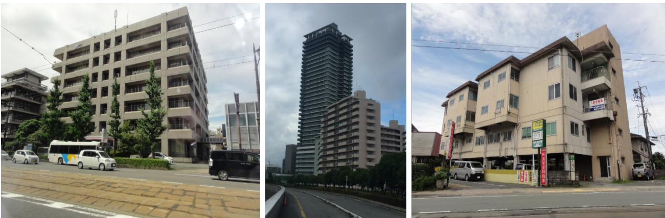
Figure 3: Example of multistory buildings with no damage.
