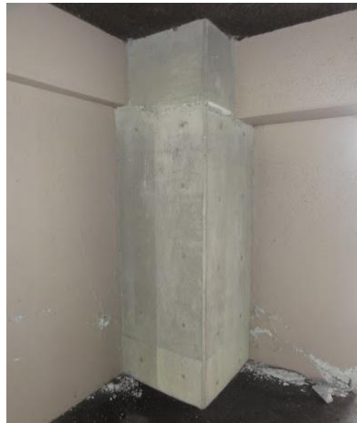
Photo 13: NW corner column and adjacent walls.
