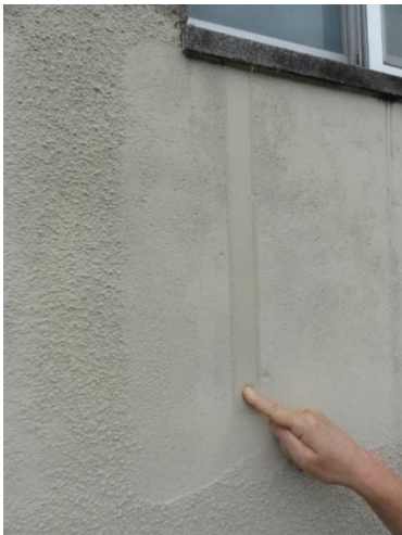
Photo 3: Separation of columns and non-structural walls as part of seismic retrofitting.
