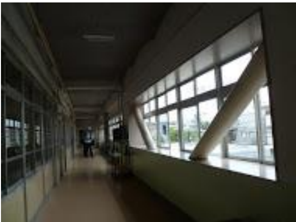
Photo 4: Interior of corridor showing retrofitted braces.
