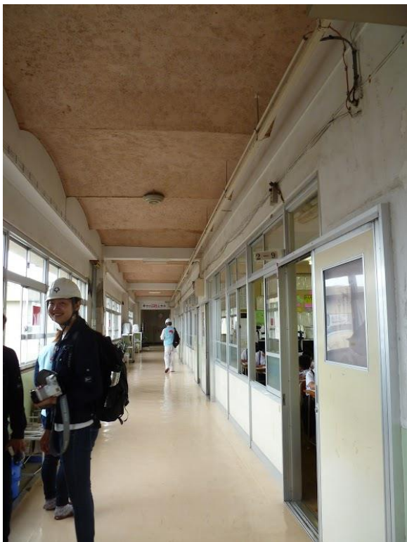
Photo 5: View of interior corridor. Interior wall of classrooms framed in non-structural aluminium joinery partitions.
