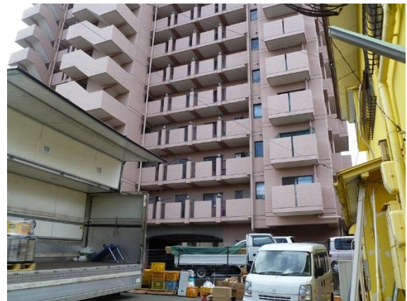
Photo 19: Apartment buildings Kumamoto. Undamaged buildings.
