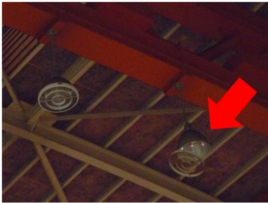
Photo 7: Building A7 detail of ceiling.
