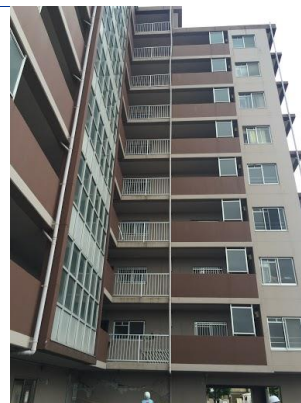
Photo 2: Building north elevation.
