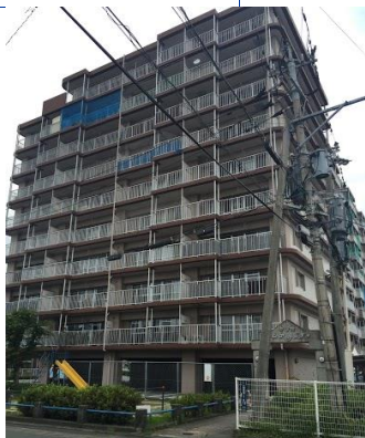
Photo 1: Building south-east elevation
