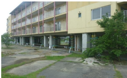
Photo 2: South-west part elevation.
