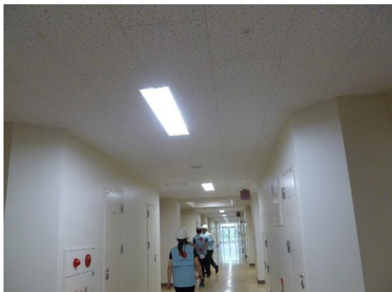
Photo 9: Building A14 building internal ceiling, no damage observed
