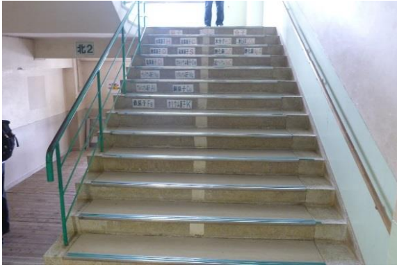
Photo 20: Building A10 no damage observed to stairs.
