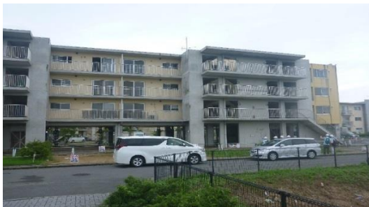
Photo 1: North-east part elevation.
