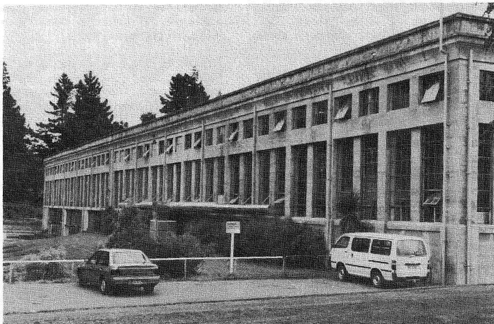
Figure 1. Lake Coleridge power station buildings (tailrace side).
