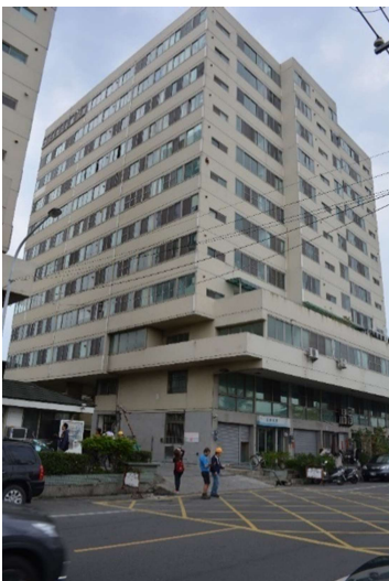
a) Front view of damage tower
