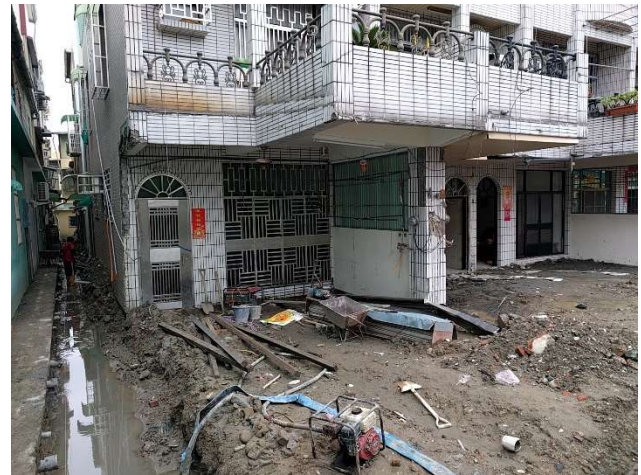
b) Site following demolition of damaged ancillary buildings
