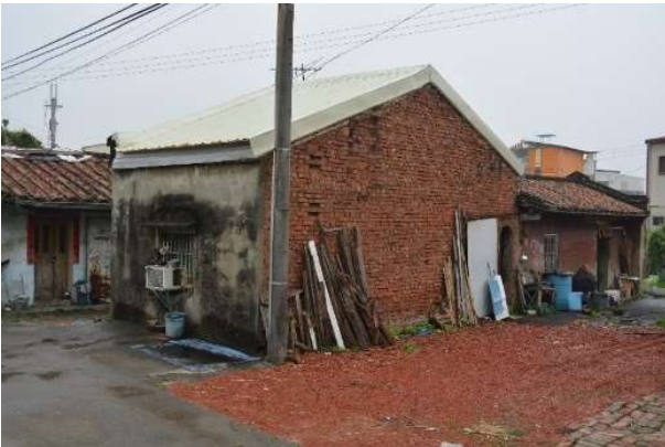
c) Repaired roof that collapsed
