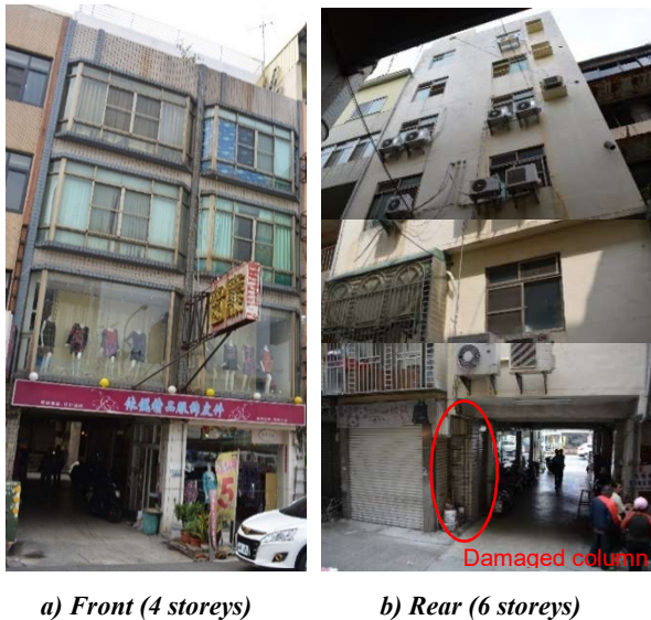
Figure 22: Added storeys on top of building.
