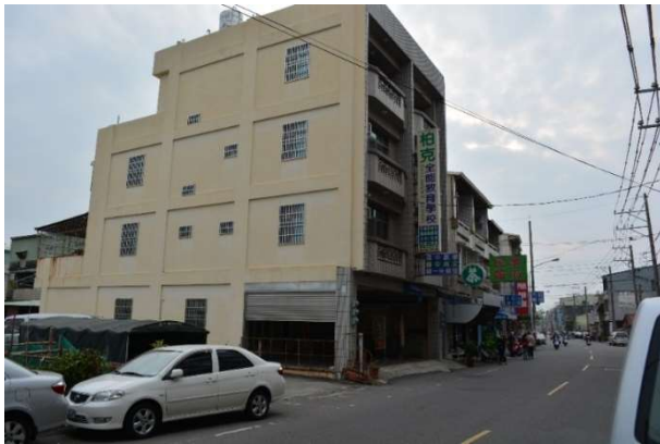
c) Modern reinforced concrete frame with infill
