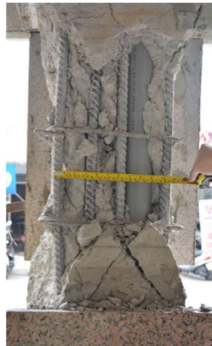
d) Downpipe, large cover, stirrup spacing
