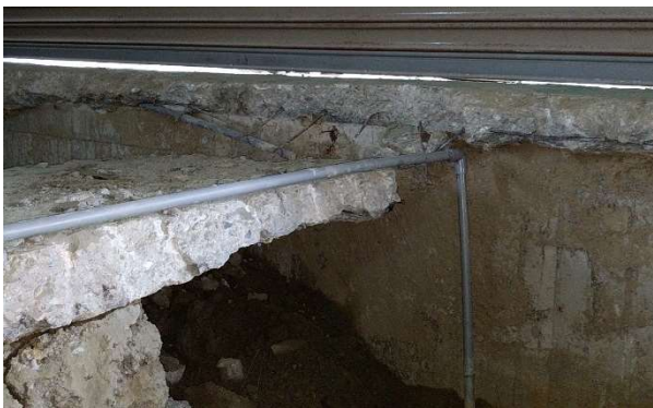
b) Pipework for dewatering
