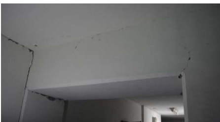
e) Coupling beams
