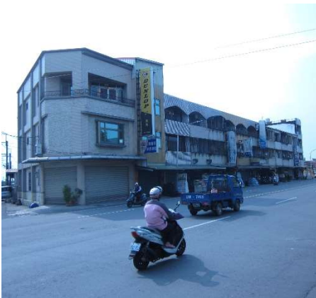
a) Overall building
