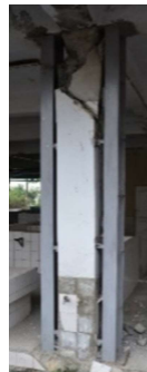
c) Column with steel supports
