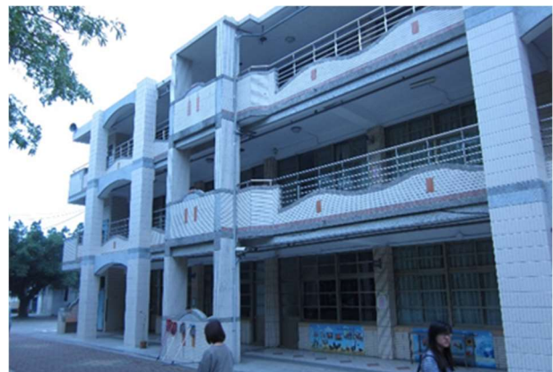
Figure 38: School building strengthened by the addition of a supplementary moment frame.
