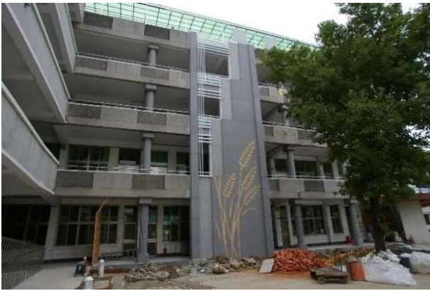
a) New concrete shear wall
