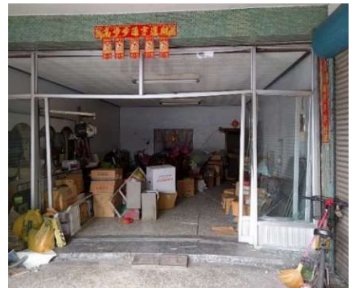
c) Hogging of floor slab
