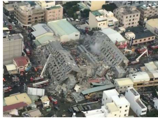
b) Weiguan Building - After (Source: www.udn.com.tw )
