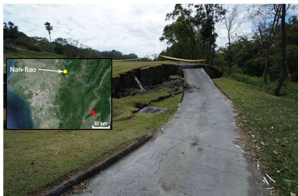
Figure 12: Slope failure at Nanbao golf course (Source: NCREE).
