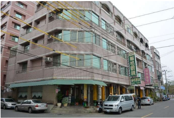
a) Overall building
