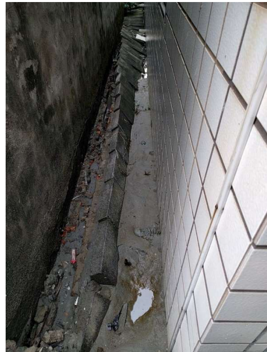
b) Drainage trench
