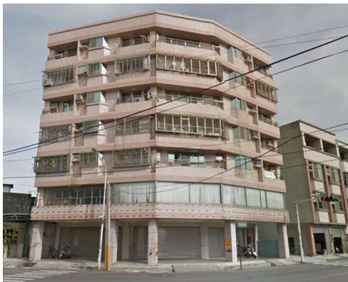
g) Xinfu Building - Before (Source: Google maps)
