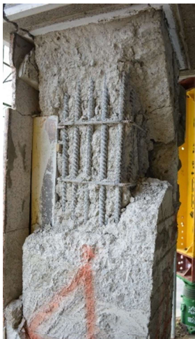
c) Electricity box, large cover, stirrup spacing
