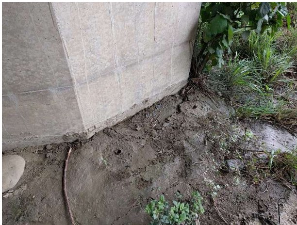
Figure 14: Ground surface settlement and crack adjacent to Freeway bridge pier on the right abutment.
