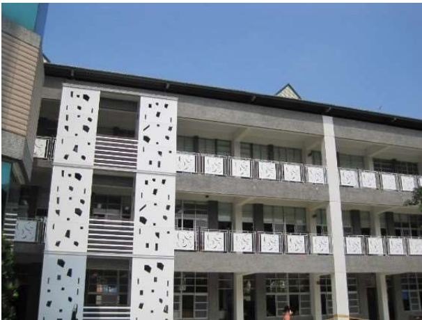
c) New concrete shear walls
