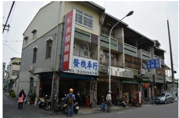
d) Original 2 storey building with additional floor
