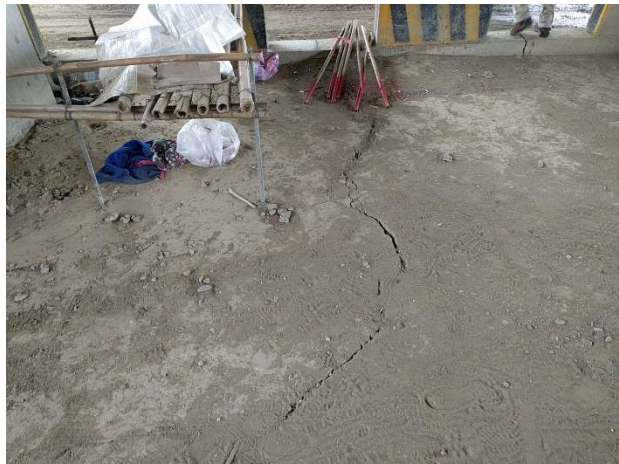
Figure 14: Ground surface settlement and crack adjacent to Freeway bridge pier on the right abutment.
