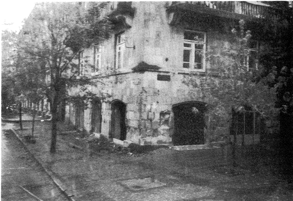
Figure 24 Building in which spread footings were being extended.
