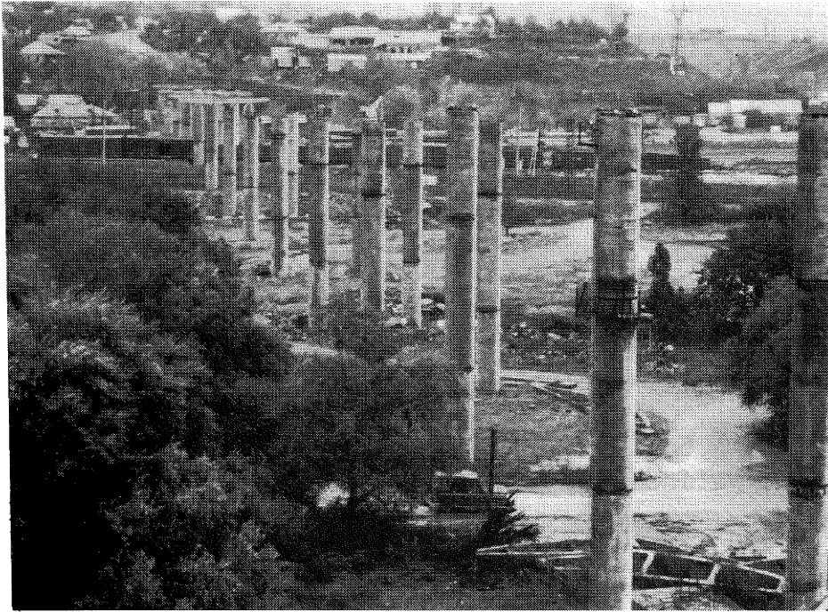
Figure 25 Precast, prestressed concrete highway bridge, under construction at Spitak at time of earthquake.
