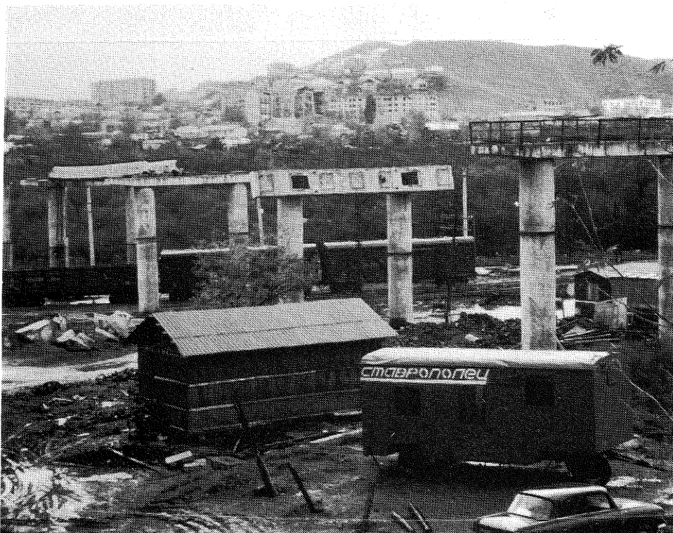
Figure 26 View of Spitak bridge, looking in the other direction.
