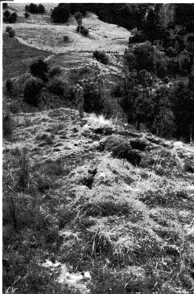
Figure 22 Damage to top of steep west trending ridge crest, 2km east of Te Karaka. Note that soil has been thrown to one side of the crack indicating a significant vertical component of movement during the earthquake.
