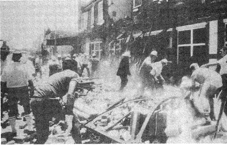
FIGURE 8 DEVASTATION AT THE KENT HOTEL, BEAUMONT STREET, HAMILTON WITHIN MINUTES OF EARTHQUAKE: AFTERMATH OF PARAPET AND AWNING COLLAPSE ONTO FOOTPATH - ALL HANDS TO THE RESCUE: (28.12.89; "NEWCASTLE HERALD")
