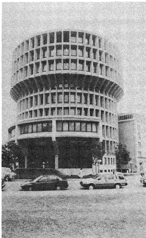
FIGURE 13 NEWCASTLE CITY COUNCIL ADMINISTRATION BUILDING AT CORNER OF KING AND BURWOOD STREETS, NEWCASTLE CBD WHICH DID NOT SUFFER ANY DAMAGE WHATSOEVER. (H.J. STUART)
