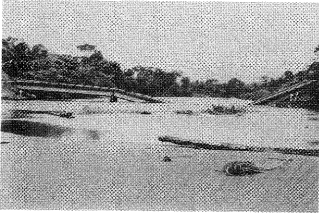
(a) General View
