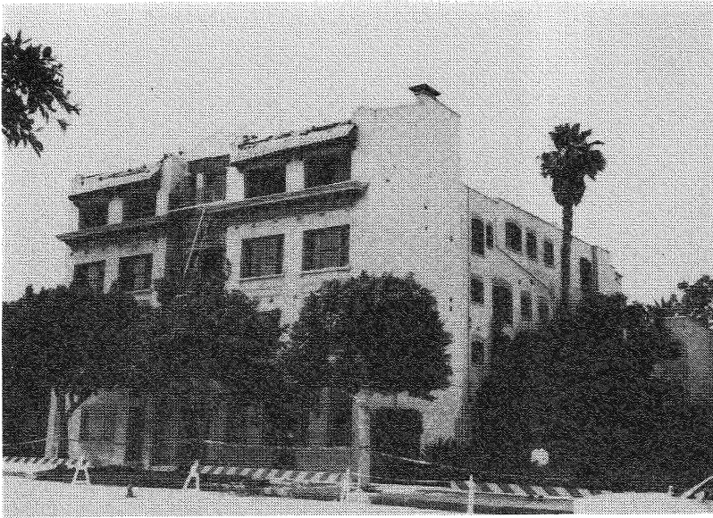
FIGURE 7. 677 COLORADO BOULEVARD, PASADENA
