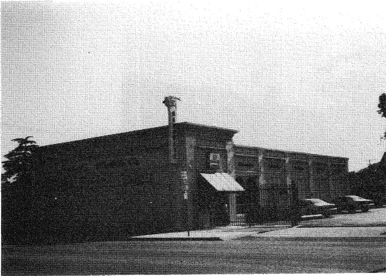
FIGURE 11. CROWN CITY HARDWARE BUILDING, 1047 NORTH ALLEN, PASADENA
