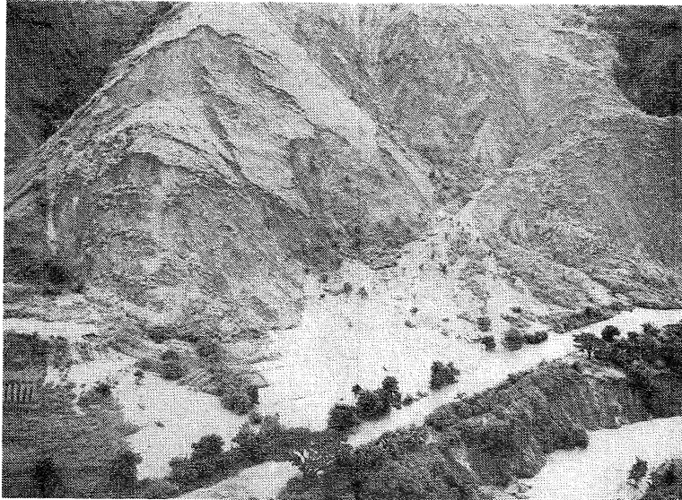
Figure 5.1.16: Dalton Pass road; landslides and mud flows obliterating houses, rice fields and roadway (Photo: Dodong Teves, PNOC)
