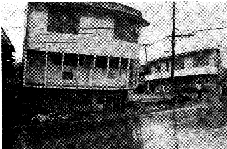
Figure 5.1.6: Dagupan City, Perez Blvd, building settlement and tilting
