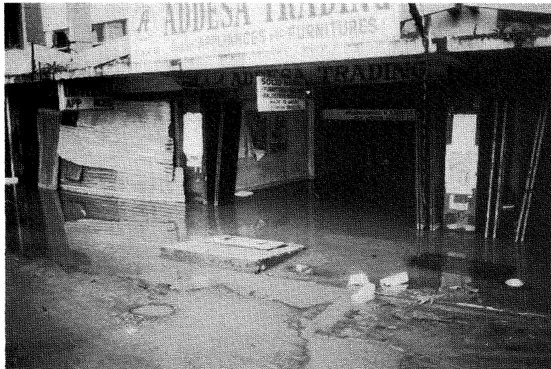
Figure 5.1.4: Dagupan City, Perez Blvd, building settlement with ground floor flooding
