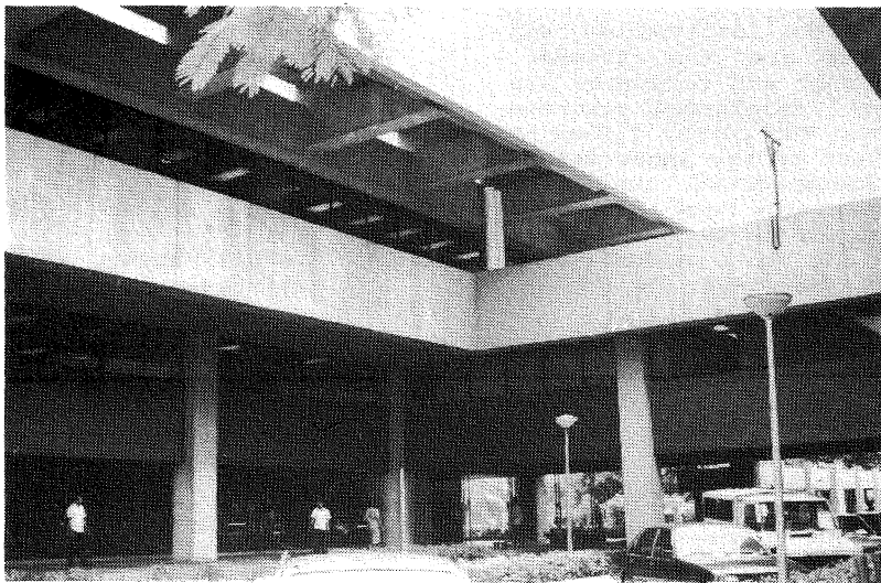
Figure C2.2: NPC Building, Quezon City; bridge structure to east wing
