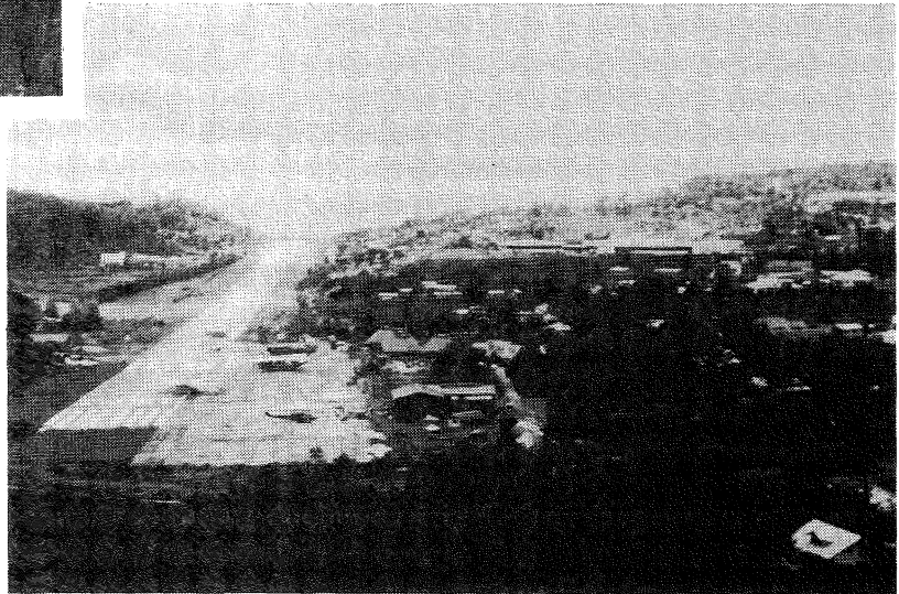
Figure 5.4.6: San Fernando Port. Damaged pier is third one along (Ian Gill, ADB)
