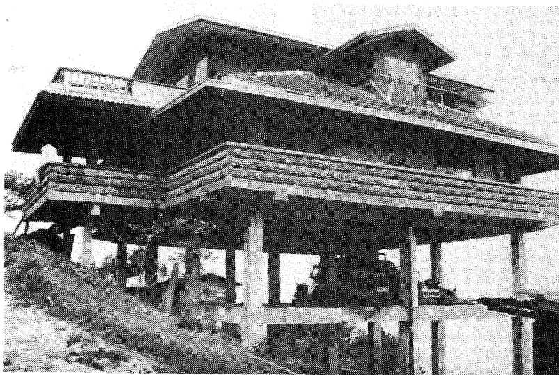
Figure 5.3.11: Notable survivor; a reinforced concrete house in Baguio. Even the balustrade is concrete, not timber
