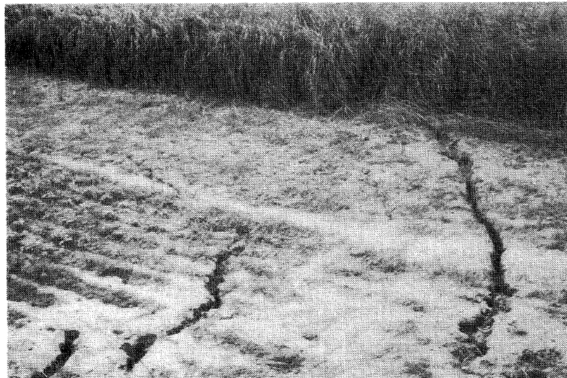
Figure 5.1.11: Fissures and ejected fine sand associated with liquefaction, Carmen Bridge (south river flood plain)
