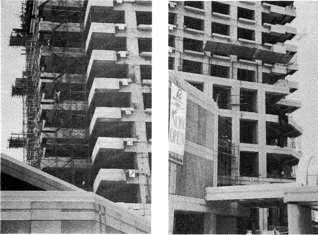
Figure 5.3.23: Multi-storey, cast insitu concrete frame, Manila
