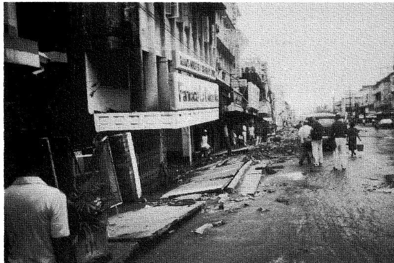
Figure 5.1.5: Dagupan City, Perez Blvd, building settlement relative to road
