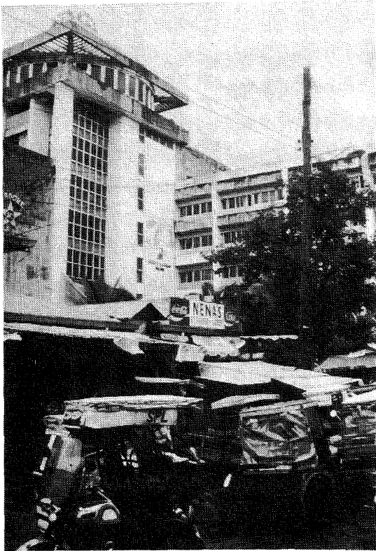
Figure 5.3.6: Deprived of sewer and water, the International Palace Hotel, Dagupan, could not operate. It was understood the building is supported on deep piles
