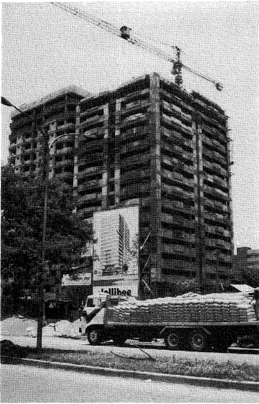
Figure 5.3.20: Multi-storey, cast insitu concrete frame, Manila
