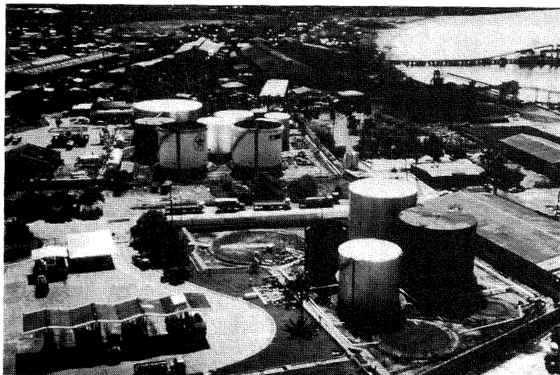
Figure C8.1: San Fernando Oil Depots (Ian Gill, ADB)
