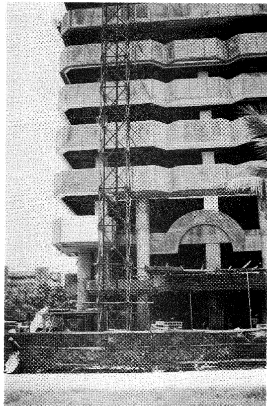
Figure 5.3.21: Multi-storey, cast insitu concrete frame, Manila
