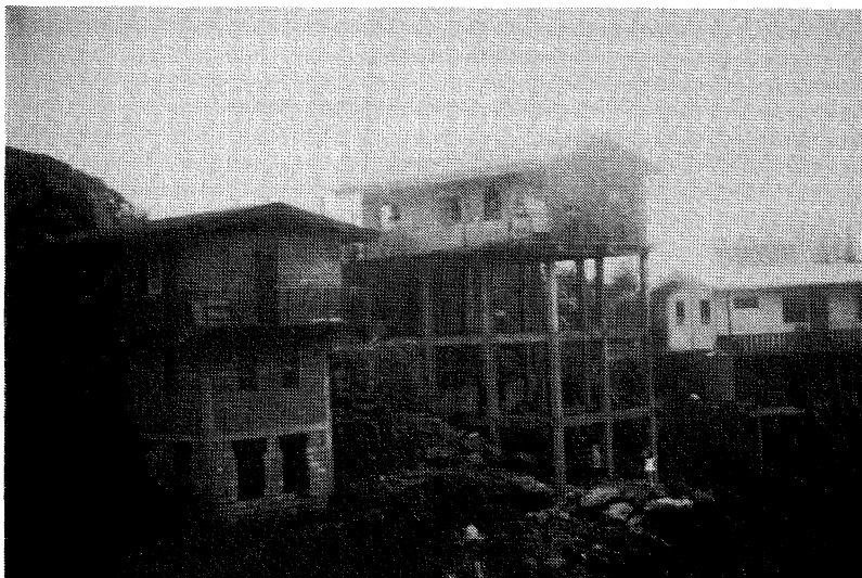
Figure 7.1.1: Baguio City; reinforced concrete frame support to house at road level
