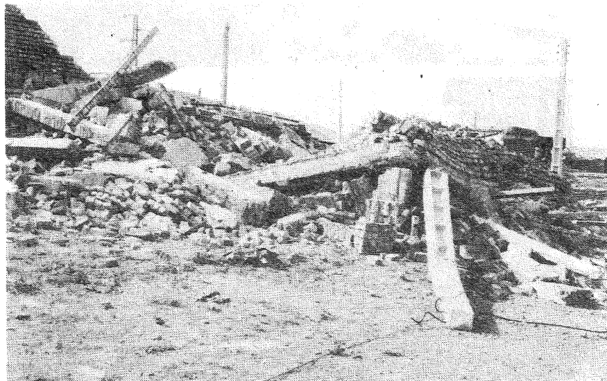
FIGURE 15: EXAMPLES OF THE DESTRUCTION IN MANJIL.
