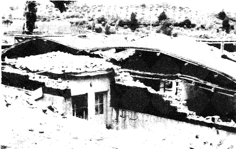
FIGURE 19: A SCHOOL BUILDING IN THE VILLAGE OF HARZEVIL TO THE EAST OF MANJIL WITH STONE WALLS AND LIGHT WOODEN TRUSS ROOF COVERED BY LIGHTWEIGHT IRON SHEETING.
