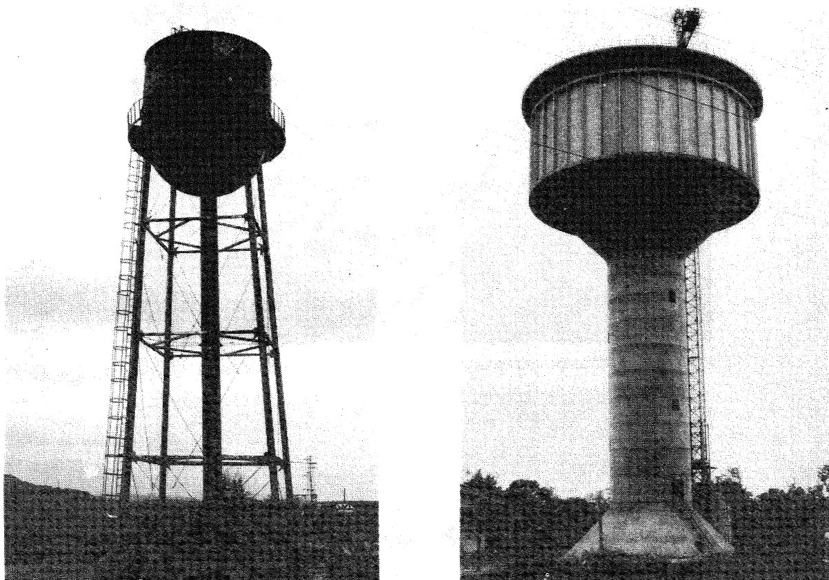
FIGURE 35: WATER TOWER IN MANJIL. THE DIAGONAL BRACINGS WERE FRACTURED BY THE EARTHQUAKE.
