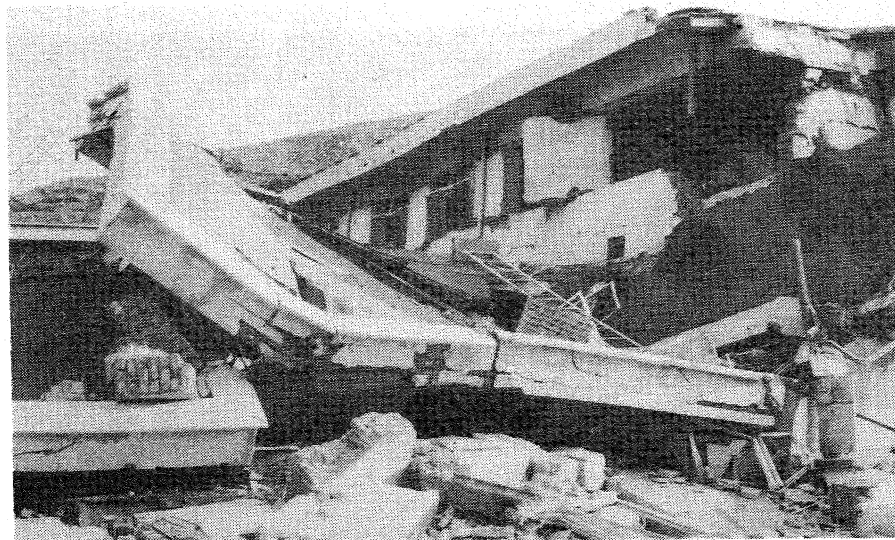
FIGURE 18: RUDBAR HOSPITAL AFTER THE EARTHQUAKE (TOP) WITH LONG CANTILEVER SPANS DAMAGED (BOTTOM).
