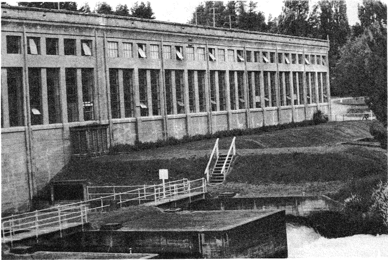
FIGURE 5. LAKE COLERIDGE HYDROELECTRIC POWER STATION.
