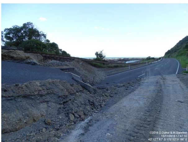
Figure 4: Example of a fault rupture on State Highway 1 that severed the East Coast fibre-optic cable. Photo: Dizhur & Giaretton.
