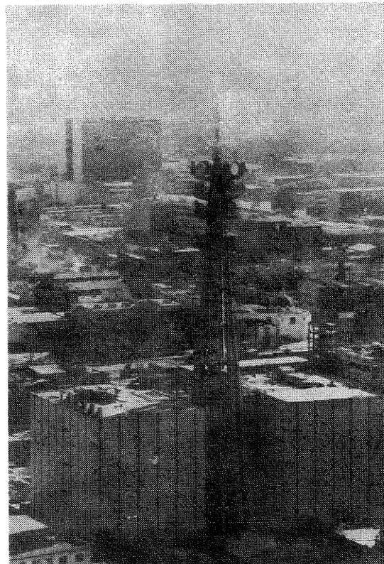
Figure 19 Telecommunications tower, Mexico City.
