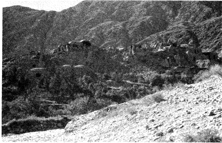
Figure 7. — Damaged village on hill.
