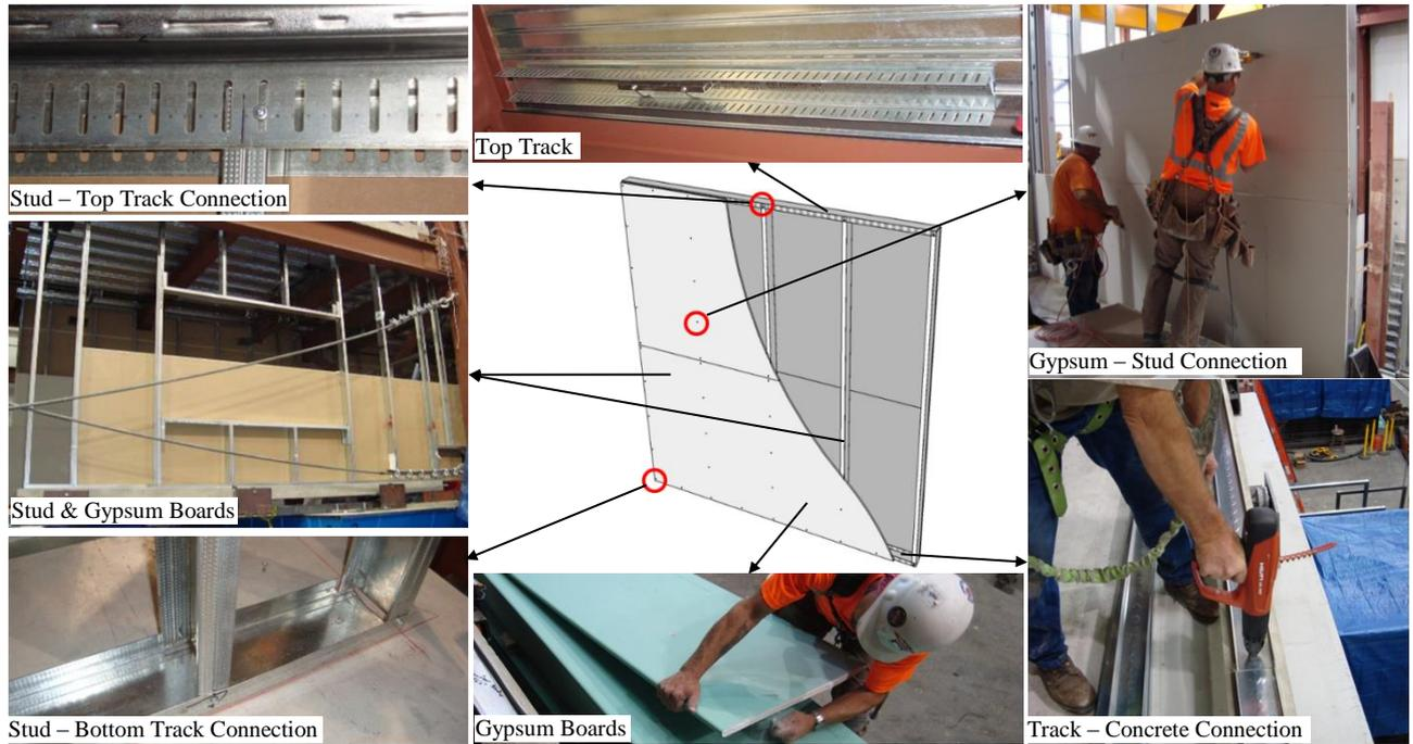
Figure 3: Typical layout and elements of a light-gauge steel-frame gypsum partition walls.
