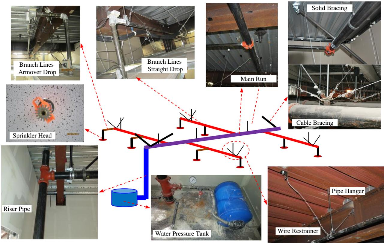
Figure 2: Typical layout and elements of a fire sprinkler piping system.
