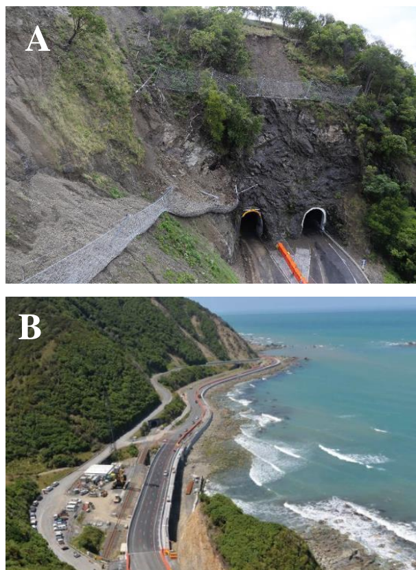
Figure 14: Examples of passive mitigation solutions implemented by NCTIR (see Figure 6 for locations). (A) Rock fall/debris catch fences protecting SH1 at the Raramai Tunnel portals, south of Kaikōura. (B) Realignment of the state highway onto the uplifted shore platform away from the hillslopes at Irongate Stream, north of Kaikōura.
