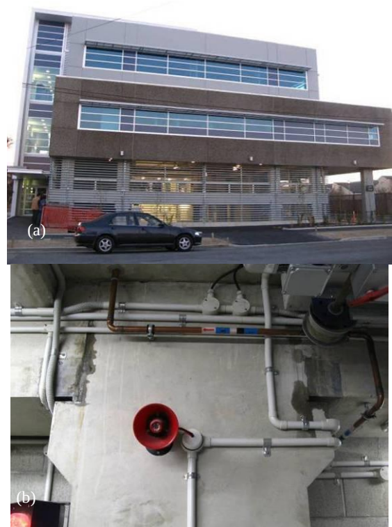
Figure 13: Self-centring precast concrete system implemented for a newly constructed private hospital facility. (Photo credit: Weng Y. Kam).
