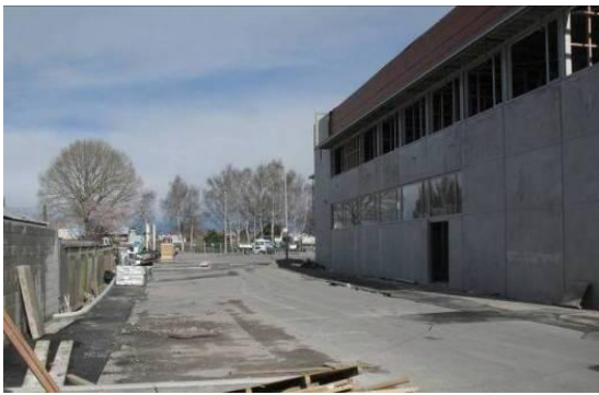
Figure 12: A tilt-up precast concrete with steel portal frames supermarket to be demolished due to differential ground settlement from liquefaction. (Photo credit: Weng Y. Kam).
