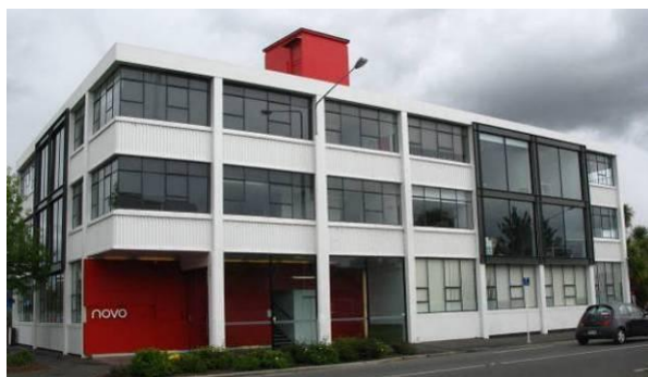
Figure 18: Seismic retrofit of non-ductile RC frames with FRP jacketing of the columns and with additional new shear walls. (Photo credit: Weng Y. Kam).
