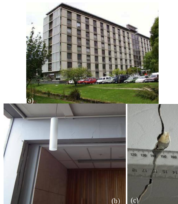
Figure 8: Beam plastic hinge of 1960s mid-rise RC building. (Photo Credit: Rajesh Dhakal).
