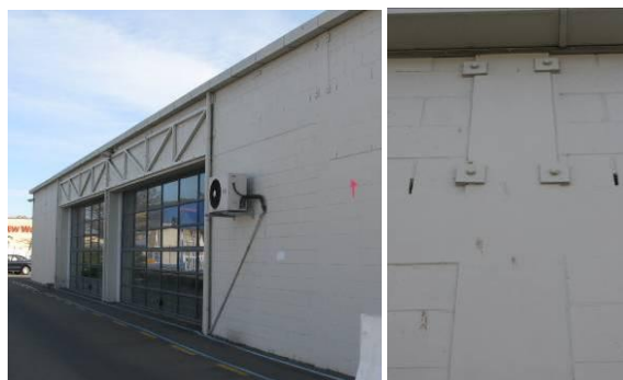
Figure 17: Infill walls parapet retrofit for infilled RC frames (Photo credit: Weng Y. Kam).
