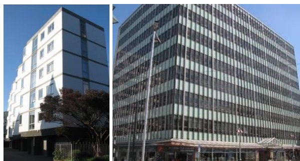
Figure 6: Mid-rise pre-1970s RC buildings with no apparent damage. (Photo Credit: Weng Y. Kam).
