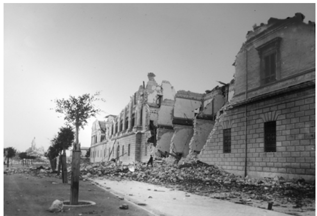
Figure 3: Destruction in the 1908 Reggion-Messina Earthquake.
