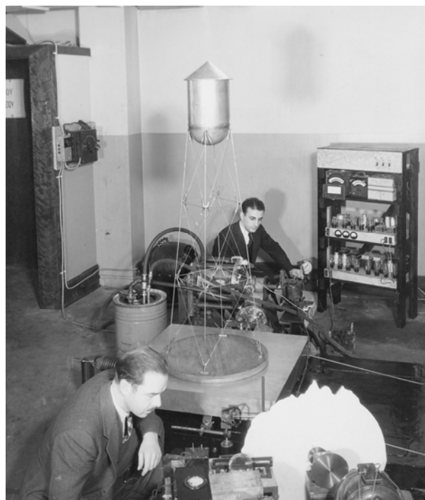
Figure 1: Arthur Ruge (foreground) conducting shake table experiments, which led to his co-invention of the electric resistance strain gauge.
