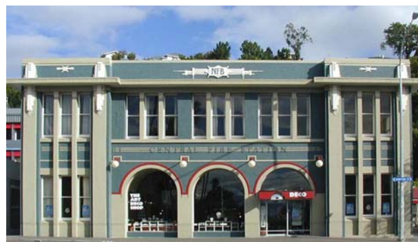
Figure 7: The current Art Deco Trust Building in Napier, New Zealand, formerly a fire station. The front portion is an exact replica, in reinforced concrete, of the unreinforced brickwork that partially collapsed in the 1931 Hawke's Bay Earthquake. The rear portion of the structure, made of reinforced concrete, survived.
