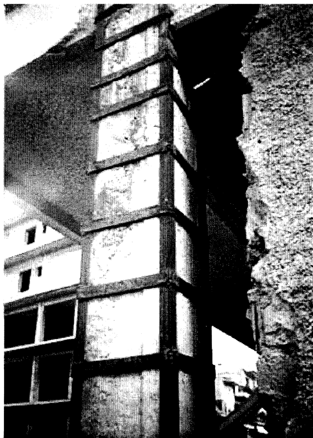
Figure 7. Construction of a steel cage around a vertical element.
