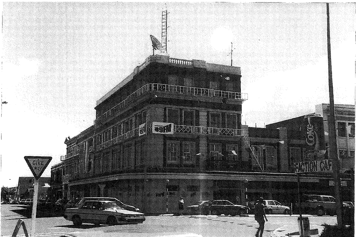
FIGURE 1 MASONIC HOTEL (built 1900-1929). First building assessed in Gisborne (1982); comprises 5 building complex; major strengthening after 1966 Gisborne earthquake
