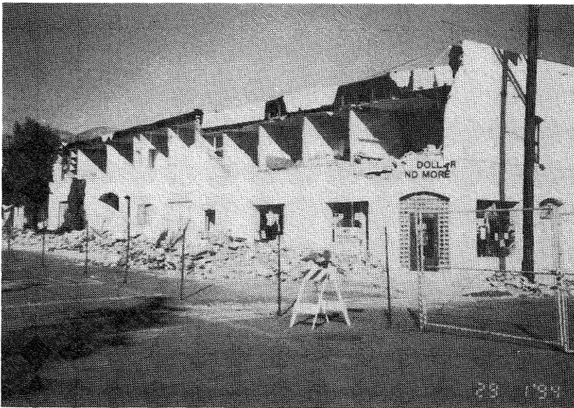
FIGURE 6.70. Unreinforced masonry structures at Fillmore, 25 miles north west of the epicentre.
