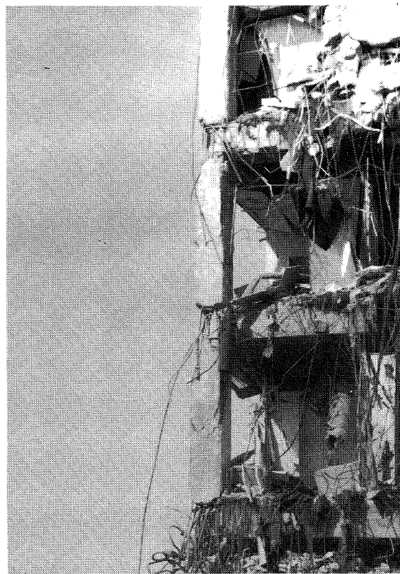
FIGURE 6.10. Kaiser Permanente, Northridge. Completely destroyed columns of Level 2 and damaged beam-column joints above.
