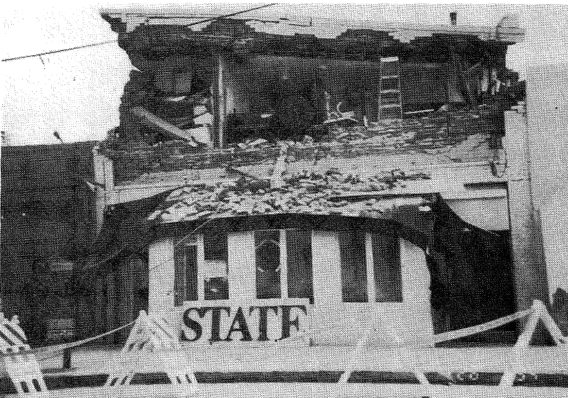
FIGURE 6.71. Unreinforced masonry structures at Santa Monica, Several small retail outlets experienced similar damage (22).
