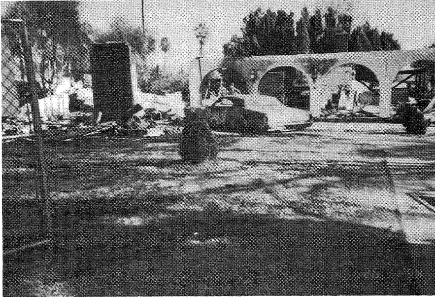
FIGURE 10.2. Gas leak initiated fire consumed this house within 20 minutes of the earthquake. It spread to and consumed an adjacent home before burning itself out (see also Figure 10.3).
