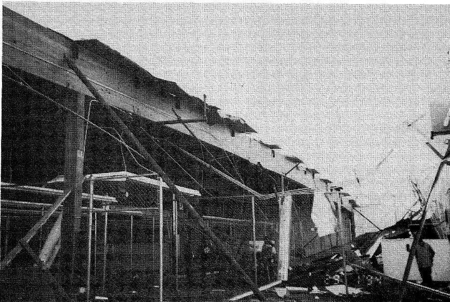
FIGURE 6.28. De Soto Drive Warehouses. Glulam portals with rafter hangers and ties prevented spread at one end only.
