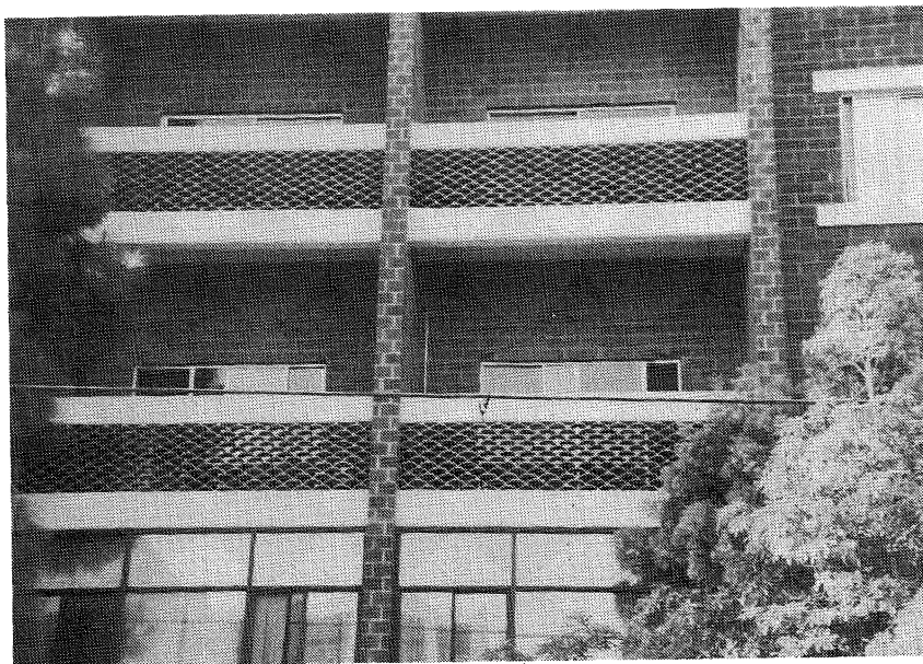
FIGURE 6.67. Berkeley East Convalescent Home, Santa Monica. 5 storey reinforced brick masonry building (21).
