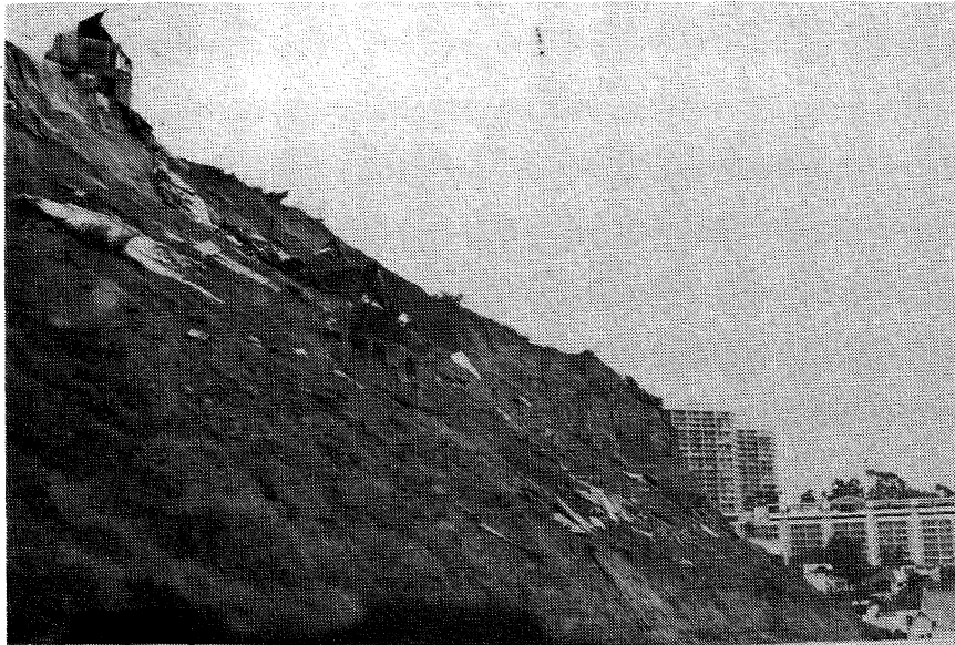
FIGURE 5.4. Landslide along the Pacific Coast Highway, Santa Monica.
