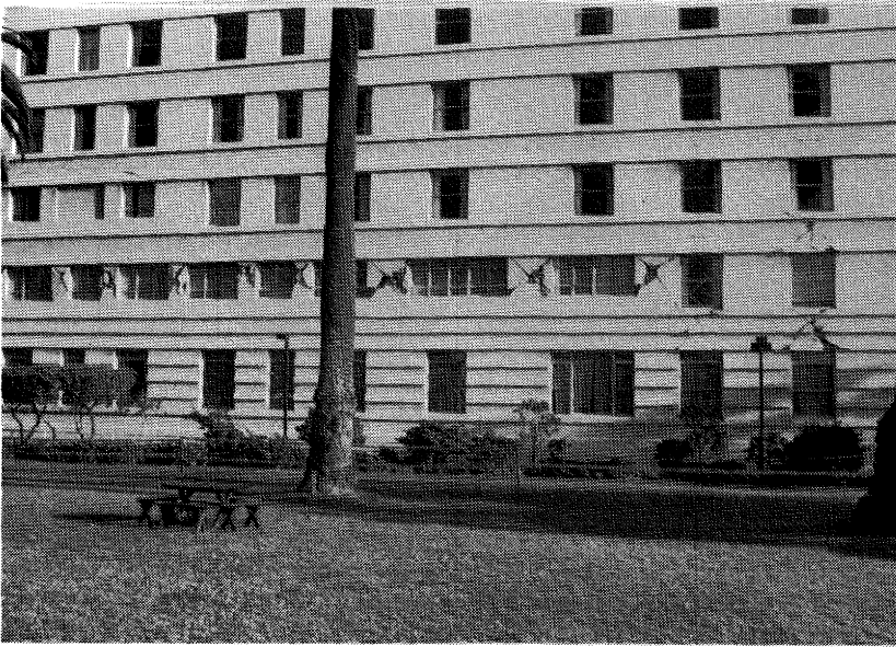
FIGURE 6.13. St Johns Hospital, Santa Monica. Elevation of the North Wing. Note: the damage to the second floor piers.
