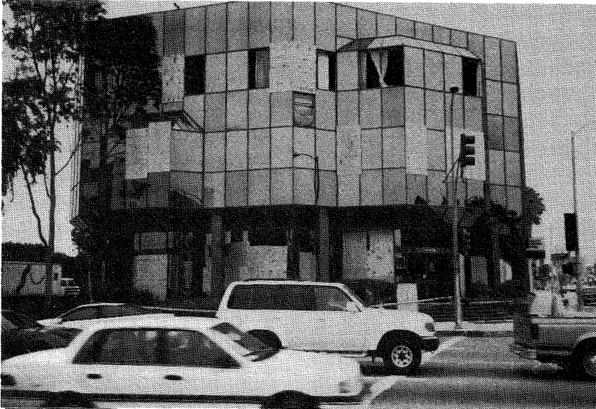
FIGURE 7.4 Medium rise office Block (4). Several glazing panels damaged particularly at changes facade plane.
