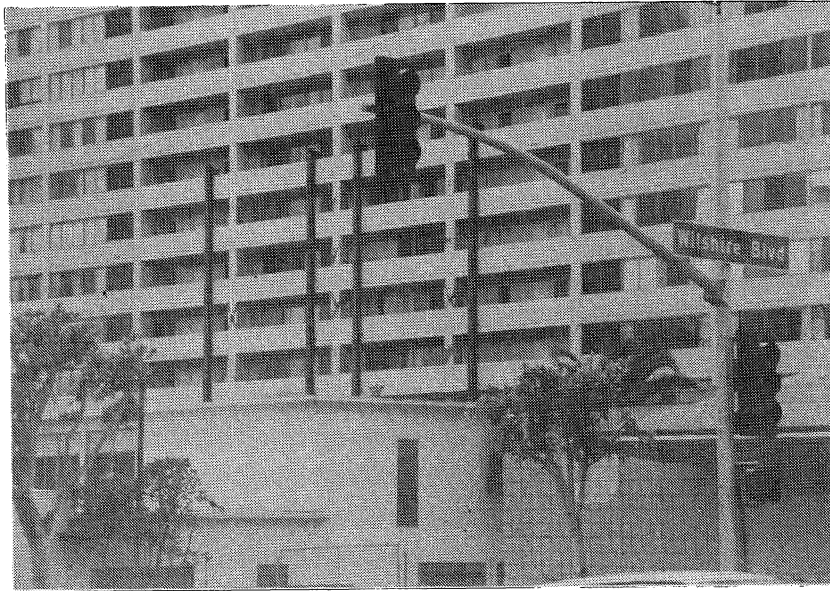
FIGURE 6.11. Champaign Tower, Santa Monica. View of east elevation of the building. Note: the extensive damage to the columns of this face.
