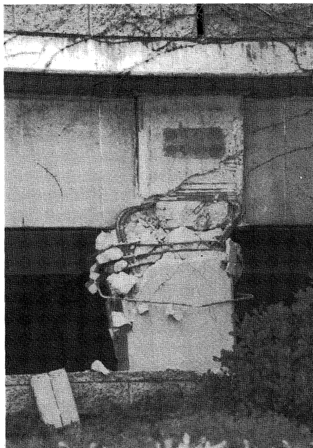
FIGURE 6.37. Sherman Oaks Galleria Car Park (south). Perimeter column at ground level.
