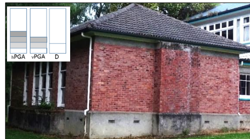
(b) Close-up of the loadbearing URM cavity-walls, Nurses' Hostel
