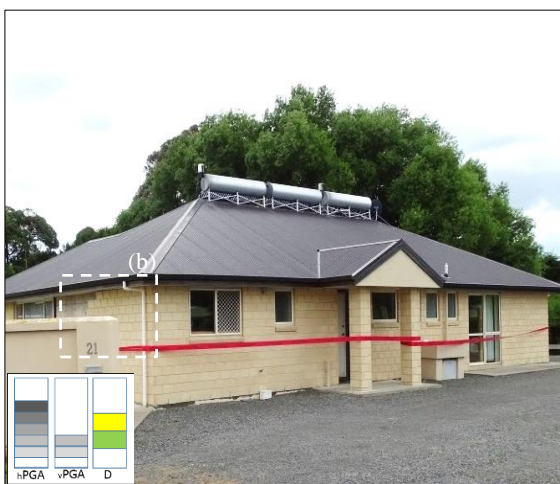
(a) Recently constructed veneer building
