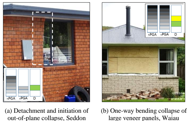
Figure 27: Examples of out-of-plane damage to veneer.
