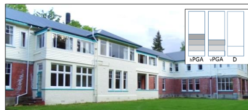
(a) Nurses' Hostel (1928-1929) with loadbearing cavity-URM walls on ground floor and timber framed walls on the upper level
