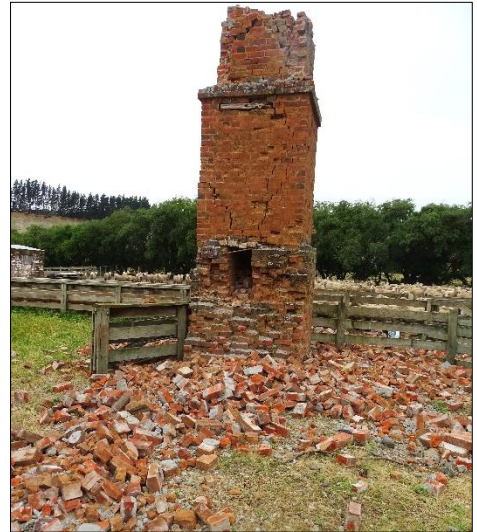
(d) Standalone historic URM chimney, located 16 km west of Seddon
