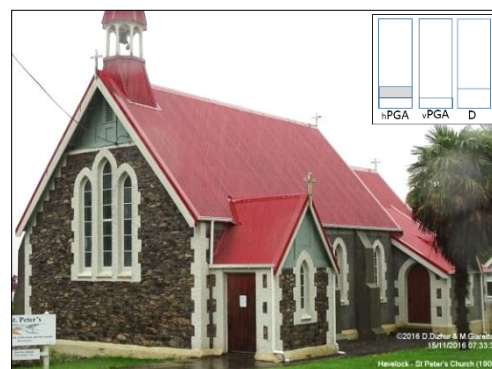
(a) St Peter's Church (1905, Heritage List #1496, likely to be seismically retrofitted)
