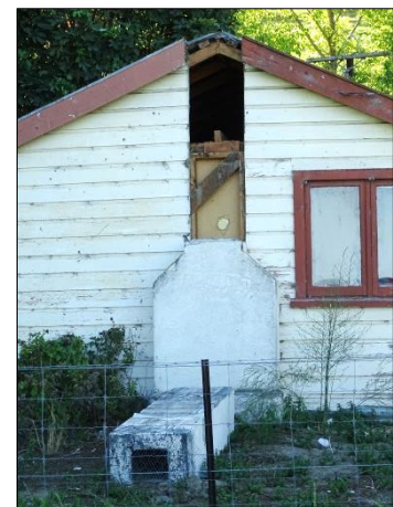
(f) Clarence, concrete stack
