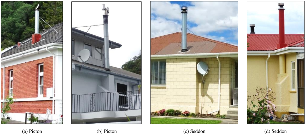
Figure 18: Examples of URM chimneys that had been removed and/or lowered to the roofline.
