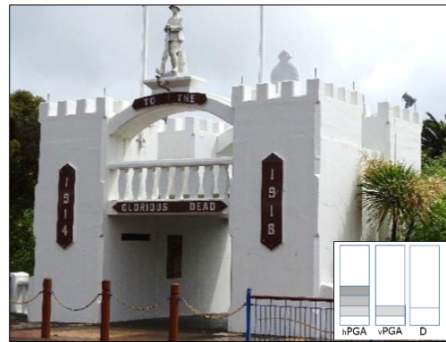
Figure 8: Vintage concrete structures in Picton (hPGA 0.262g, vPGA 0.100g – QCCS).
