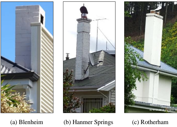
Figure 23: Examples of tall non-damaged URM chimneys.
