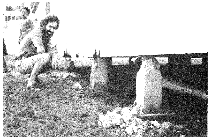
Fig 6. Damage to concrete House piles Niusawa High School
