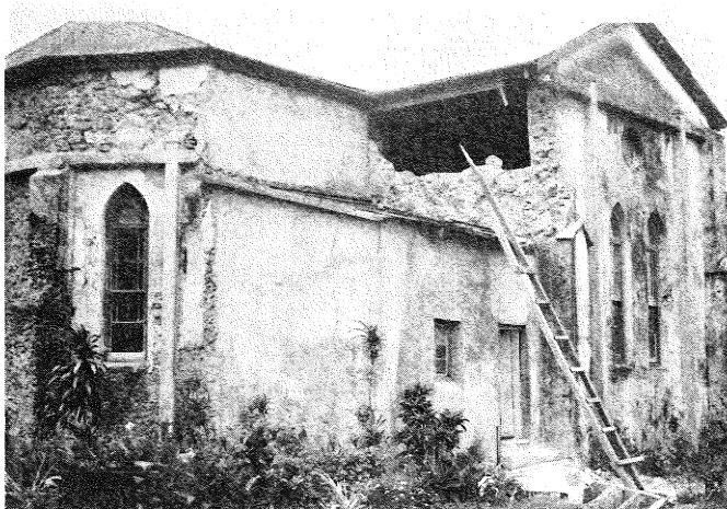
Fig. 15 Failure of rubble concrete - Napuka Catholic Church (Note Strengthening)
