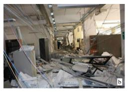
Figure 1: (a) Collapsed suspended ceilings and (b) gypsum block partitions [2].
