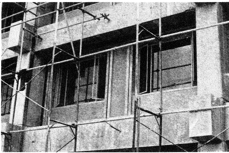
FIGURE 11: EXTERIOR CLADDING ELEMENTS ARE POSITIONED INSIDE EXTERNAL FRAME RESULTING IN SIMPLER AND MORE EFFECTIVE SEPARATION DETAILS
