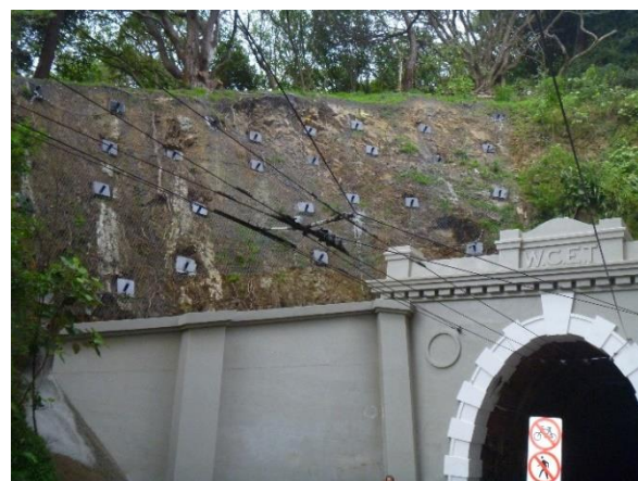
Figure 11: Rockfall protection mesh installed above the Hataitai end portal. View of the finished portal walls.
