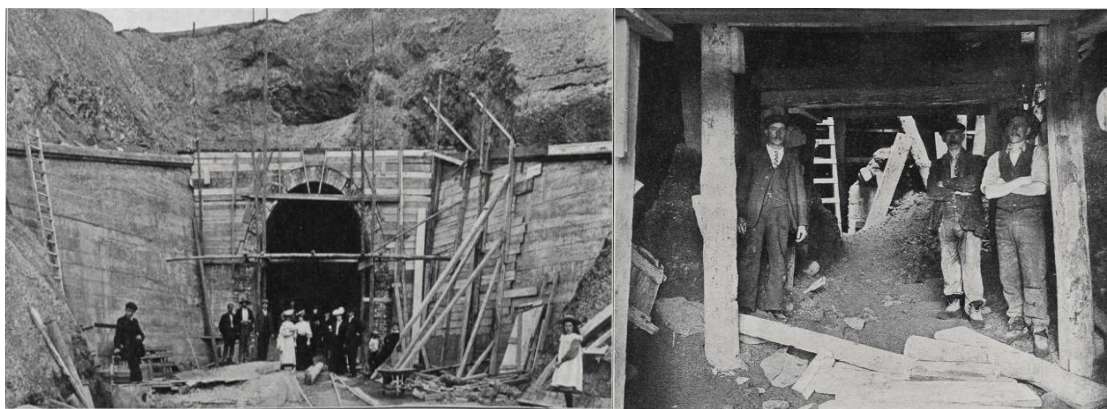
Figure 4: Photographs of the construction of the portals (left) and tunnel section (right) of Hataitai tunnel taken in 1907. The photograph of the tunnel section is following a roof failure [10].
