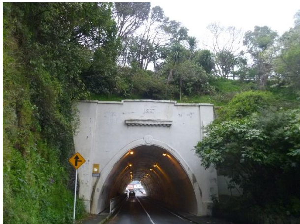
Figure 16: View of the south portal of Northland tunnel. 10 m to 15 m high and steep rock slope at the left-hand side of the portal (photograph before the strengthening works).
