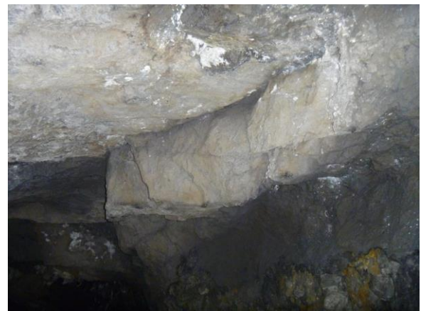
Figure 8: Wedge failure mechanism observed on the roof of Orongorongo water supply tunnel in the Wellington Region.
