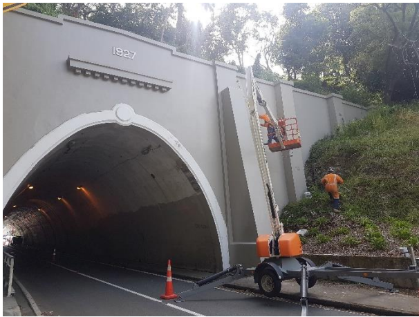
Figure 20: South portal and wing walls post construction of the strengthening measures – Northland tunnel.
