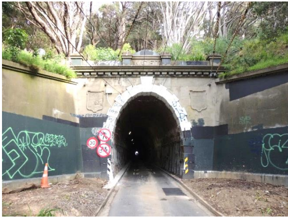
Figure 9: Hataitai Bus tunnel west portal, parapet and wing walls (before the strengthening works).
