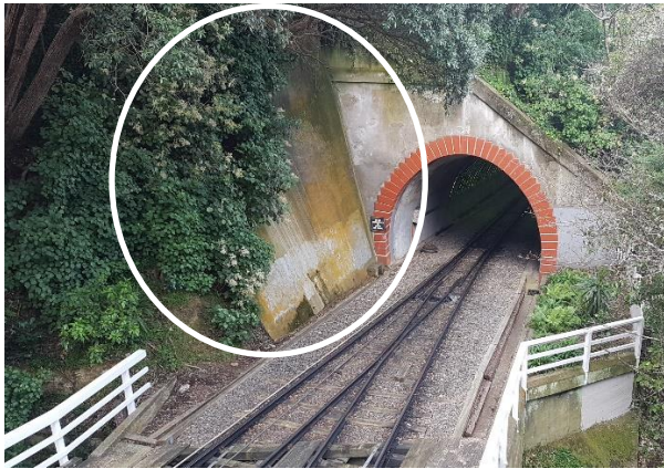
Figure 34: Unreinforced concrete facing on the slope face at the north side of the upper portal of the middle tunnel.
