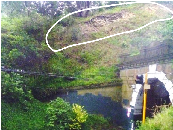
Figure 10: Rockfall hazard from slope above the east portal of the Hataitai Bus tunnel (rockfall source shown in white).
