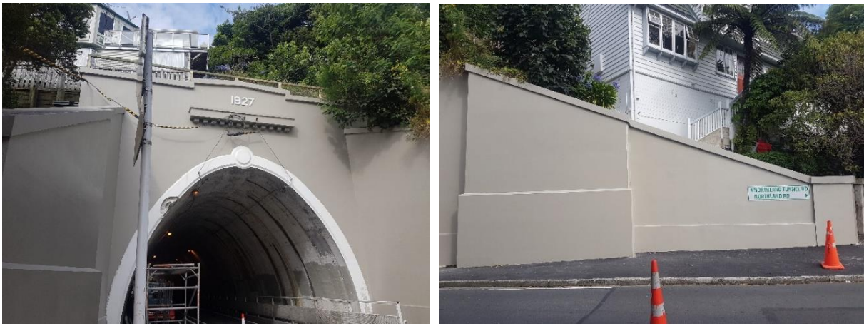
Figure 17: North portal and wing walls after strengthening – Northland tunnel.
