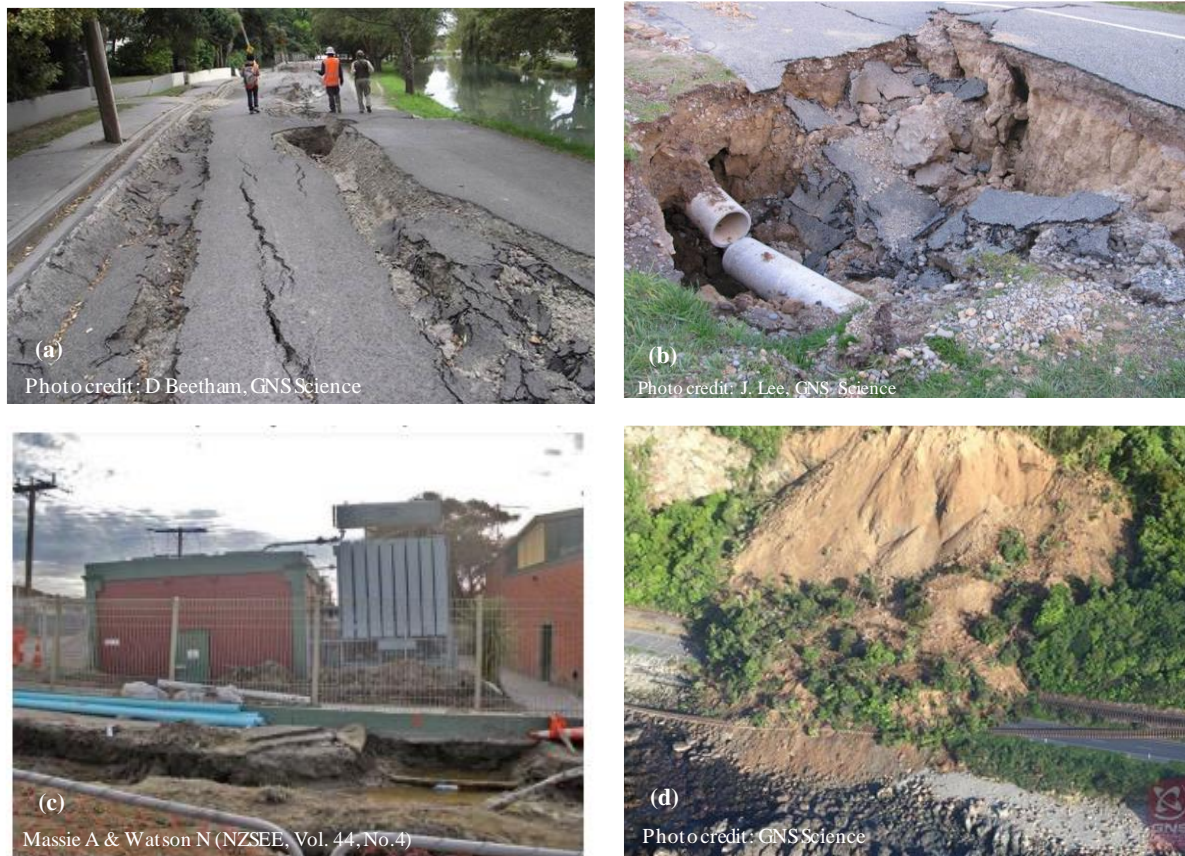
Figure 1: Examples of damaged infrastructure network assets from the 2010-2011 Canterbury earthquakes (Figures a-c) and the 2016 Kaikōura earthquake (Figure d).
