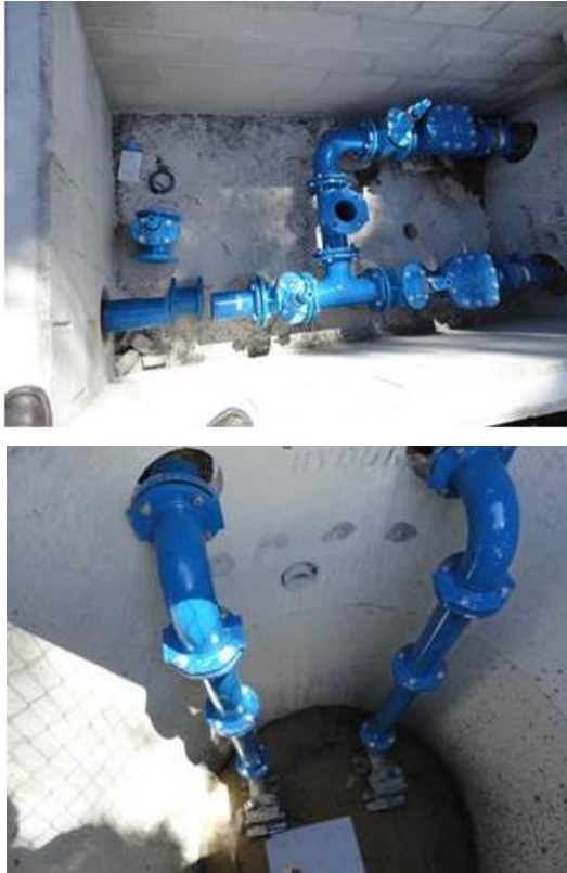
Figure 8: Two types of chambers (square and circular) in submersible pump station. (Photos courtesy: RLC).
