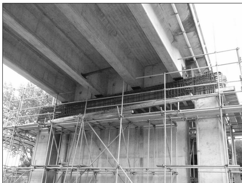
Figure 10. Strengthening frame under construction alongside existing pier.
