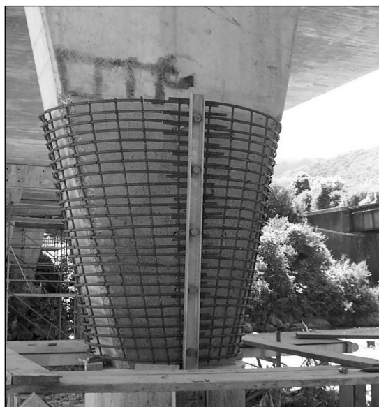
Figure 4. Reinforcement in concrete jacket.
