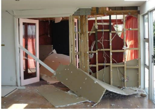
Figure 38: A severe failure of the plasterboard internal linings after the 2011 Christchurch [5].
