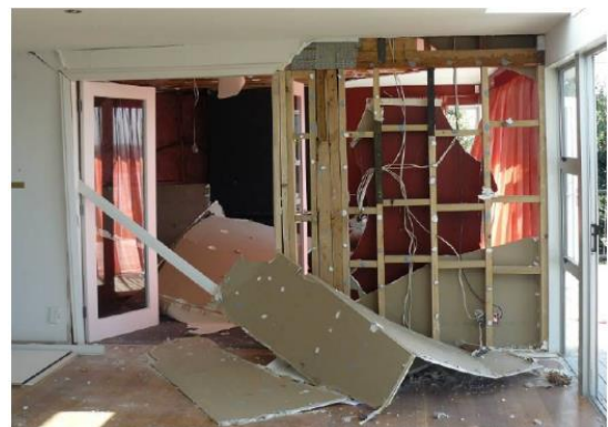
Figure 37: A severe failure of the plasterboard internal linings after the 2011 Christchurch [5].
