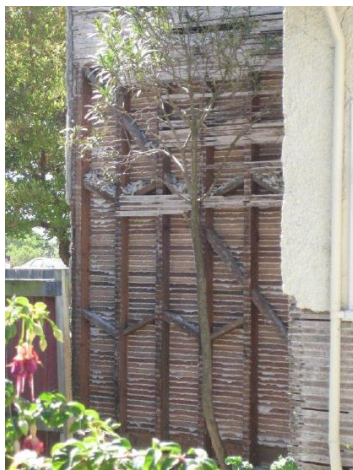
Figure 3: A failure example of lath and plaster wall [5].
