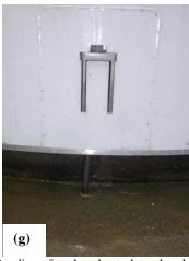
Bending of anchor due to lateral tank movement relative to plinth
