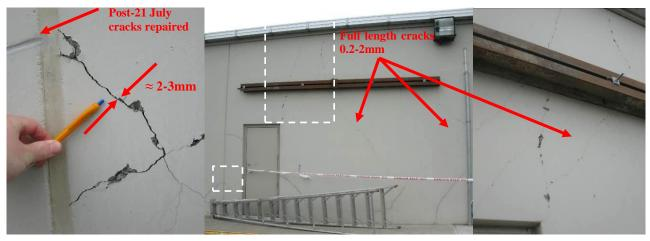
Figure 14: Precast concrete wall panels damaged following the 16 August earthquake. The panels had previously been repaired by epoxy injection of cracks following the 21 July earthquake.
