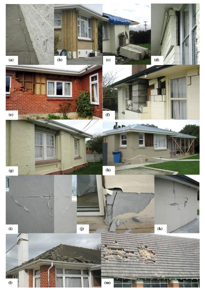
Figure 12: Various observations for residential buildings: (a) minor foundation cracking; (b) stabilisation of cladding after the 21 July event; (c) chimney collapse; (d)-(h) collapse of brick veneer at roof soffit, around chimneys, between openings; (i)-(k) cracking of plaster coating, and; (l)-(m) detachment and falling of roof tiles on churches and housing.
