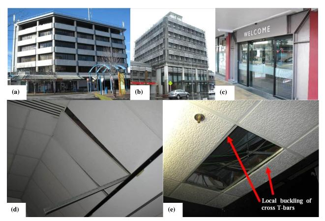
Figure 16: The largest commercial buildings in the Blenheim CBD: (a) Porse House; (b) Rangitane house. (c) One of several twostorey buildings retrofitted earlier in 2013. Observed failure of ceiling system grid members due to: (d) rivet connection failures; (e) local buckling of grid members resulting in falling tiles.
