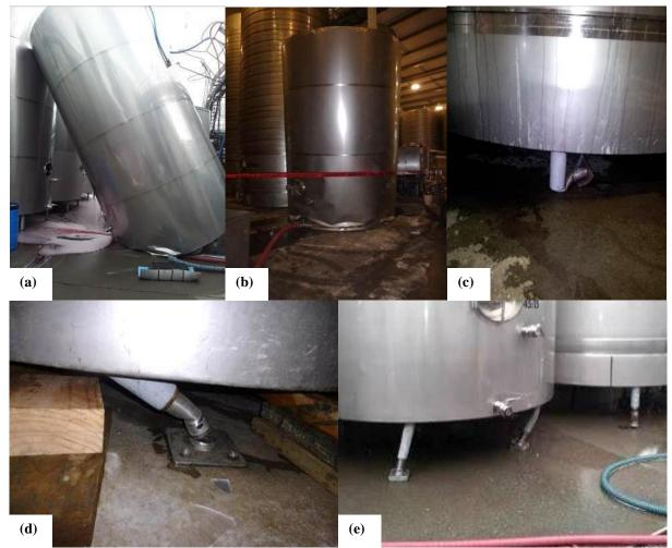
Damage to leg mounted tanks following buckling failure of tank legs
