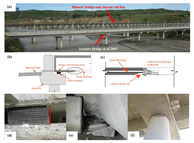
Figure 4: (a) The 275 m Awatere Bridge; (b) details of the abutment-diaphragm connection; (c) post- 21 July damage at north abutment. Post-16 August damage; (d) rubber bearings indicate residual longitudinal displacement; (e) spalling of cover concrete at edge of U-bream girders and; (f) spalling at central piers (last image courtesy of NZTA [13]).
