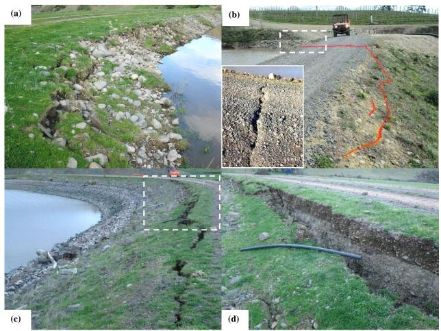
Figure 11: Various damage observations to water storage dams: (a) movement of riprap on the upstream shoulder of Dam A; (b) longitudinal and transverse crack (inset) to the crest of Dam I; (c)-(d) extensive damage at Dam E included longitudinal cracking to the full crest length.
