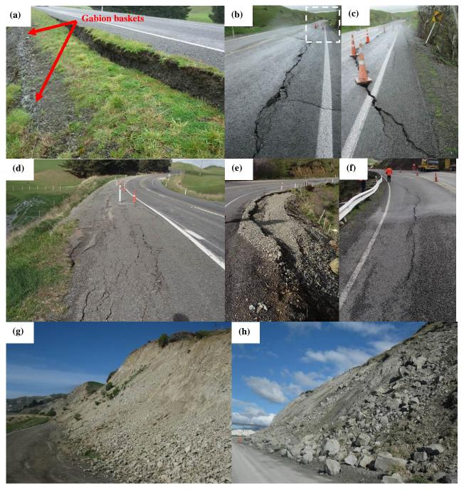
Figure 3: (a)-(d) Damage to State Highway 1 indicates instability of engineered fill materials and shoulders; (e)-(f) similar damage on Weld Pass; (g)-(h) slips on local roads within 1 kilometres of the earthquake source (Photos (d-f) courtesy of NZTA).
