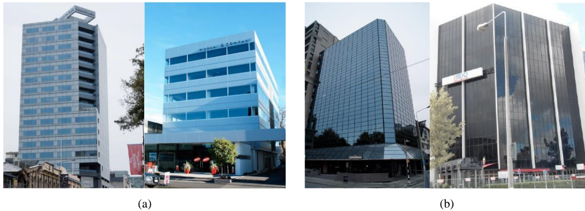
Figure 2: Typical example of glazing cladding systems [1]; (a) curtain wall, and (b) stick curtain.
