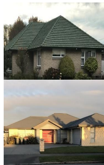
Figure 4: Typical example of masonry veneer cladding system.
