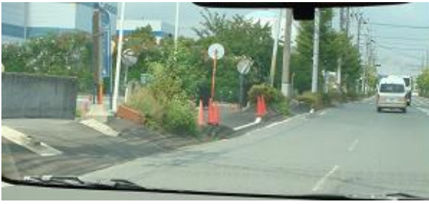
Figure 8: A section of the road which underwent settlement as a result of liquefaction.
