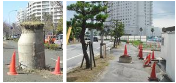
Figure 10: (a) A manhole uplifted by as much as 2 m (photo by I. Towhata); (b) several manholes protruding up from a street in Urayasu.
