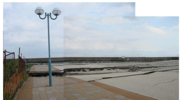
Figure 11: Longitudinal cracks at the backfill of the quay wall due to lateral movement of the wall towards the bay.
