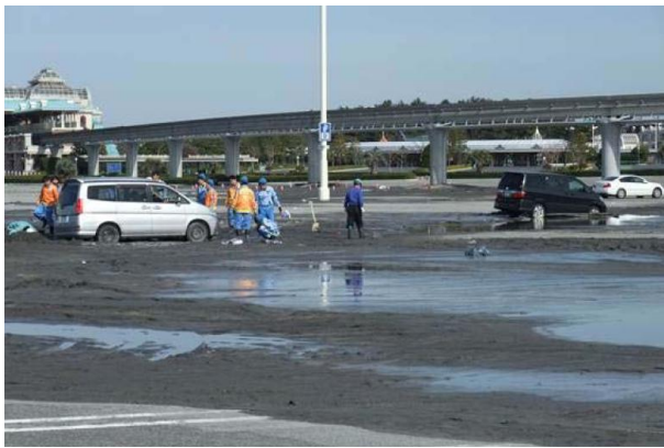
Figure 13: Parking areas in Tokyo Disney Resort covered by sand boils (Photo by S. Yasuda).
