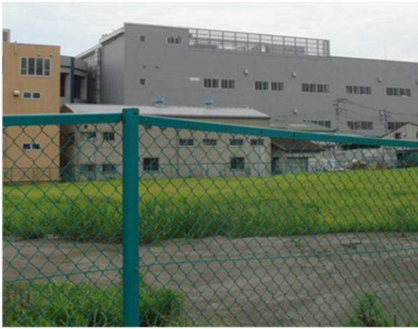
Figure 19: An undamaged building resting on improved foundation ground. Adjacent to it, sand boils were visible everywhere.
