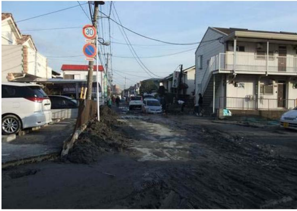
Figure 12: Residential houses in Hinode, Urayasu City land covered by ejected sands immediately after the earthquake (Photo by S. Yasuda).
