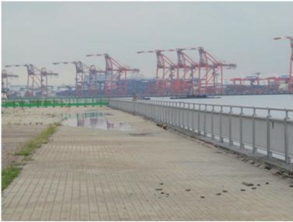
Figure 16: Lateral displacement of sheet pile quay wall in Shiokaze Park and associated deformation of the backfill.
