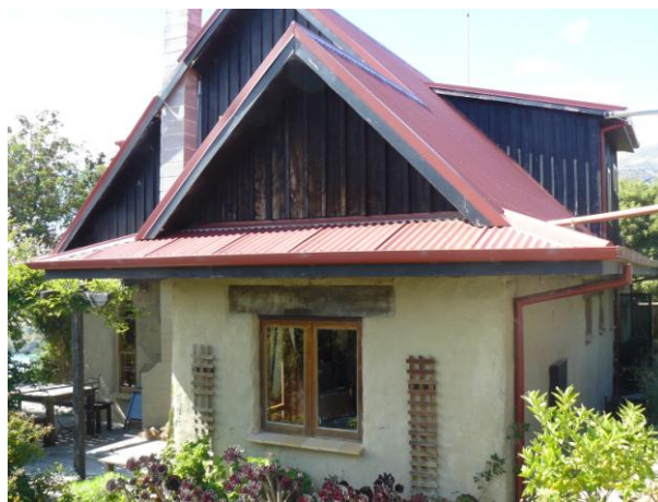
Figure 15: Diamond Harbour reinforced adobe house overall view.
