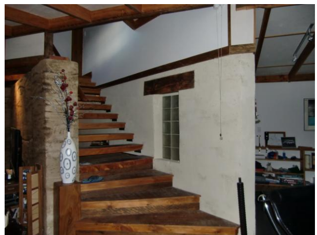
Figure 22: Little River rammed earth House 19 internal feature wall and stairway. (Photo G North)
