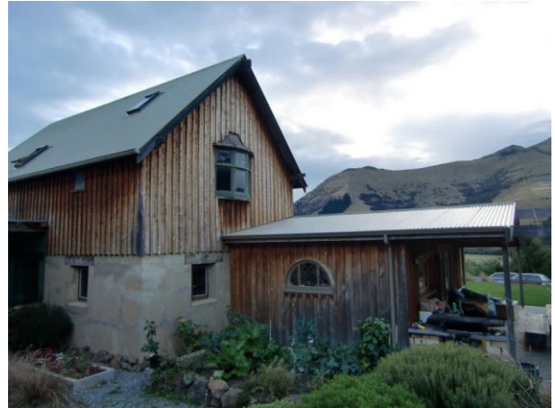
Figure 20: Little River rammed earth house 19 overview showing exterior rammed walls.
