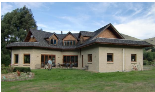
Figure 24: Little River pressed earth house 18 overview of north facing walls.
