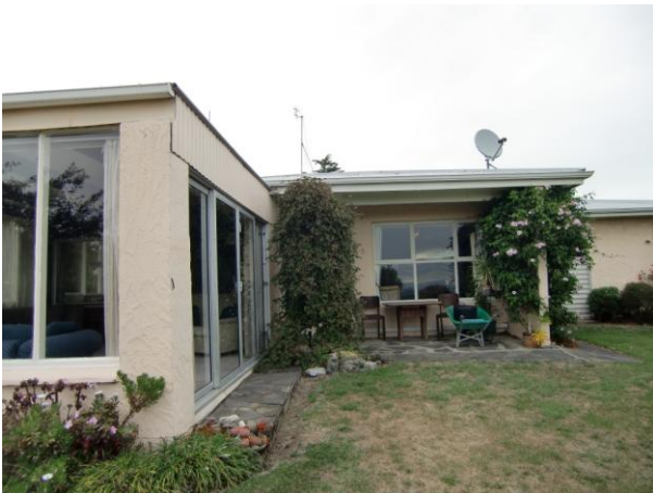
Figure 8: Unreinforced Rammed Earth Kennedy's Bush Road (Building 23) showing overall layout. New conventional addition to left front.
