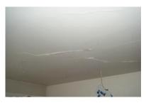
(c) Plasterboard cracks in a 2-storey residential house
