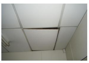
Damage to flange of the grid beam due to tile impact
