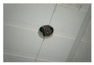
Rigid sprinkler with sufficient gap: no extra damage due to ceiling-sprinkler interaction
