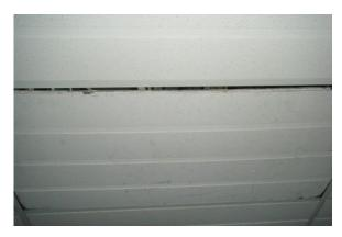
Dislocation of ceiling tile due to vertical acceleration
