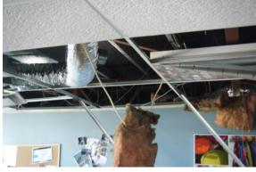
Ceiling damage caused by unbraced AC ducts
