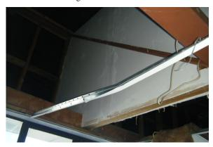
Breaking, buckling and twisting of grid members due to large compression force
