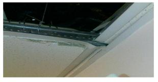
Damage to grid members due to excessive compression force (Photos: K Hogg)
