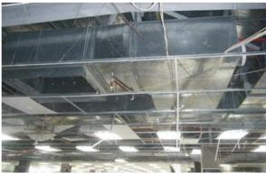
Damaged ceiling with inadequate service height
