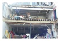
(b) Different extent of ceiling damage in different floors of a damaged building
