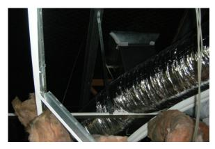
Failure of grid cross-member connection
