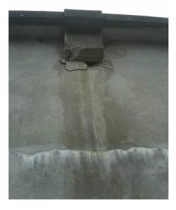
Figure 10: Upper Balmoral Reservoir – concrete damage at roof beam wall support.
