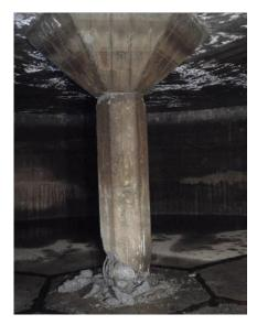
Figure 7: Clifton 3 – internal column failure.
