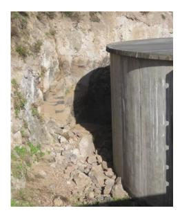
Figure 6: McCormacks Bay No.1 Reservoir – rock fall behind reservoir.
