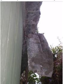
Figure 8: Clifton 3 – failure of roof overhanging nib (repaired nib shown).
