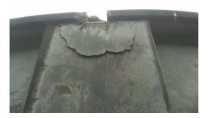
Figure 9: Upper Balmoral Reservoir -concrete shear failure at pilaster locations due to roof beam (concealed) impact.
