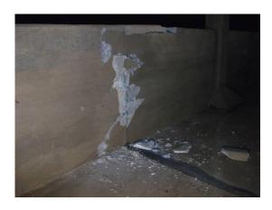
Figure 3: Huntsbury No.1 Reservoir – dividing wall failure.
