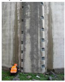
Figure 5: McCormacks Bay No.1 Reservoir – leaking vertical construction joints.
