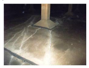
Figure 2: Huntsbury No.1 Reservoir - base-slab cracking.
