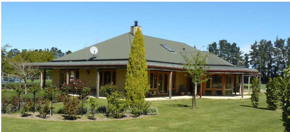
Figure 10: Charing Cross Adobe House (Building 4) 1999. Located between the epicentre and major fault rupture. Reinforcing similar to that specified in the NZ Earth Building Standards. Minor cracking mostly due to differential ground movement.
