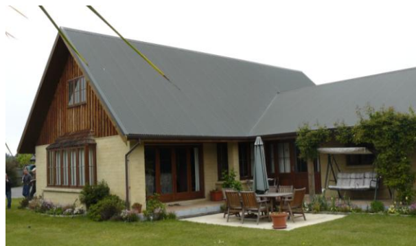
Figure 14: Spencerville Light Timber Frame House with Cinva Pressed Earth Brick Veneer (Building 11a).
