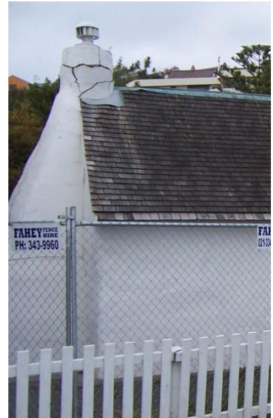
a) Lower parts of walls made of sod, upper walls predominantly cob, cement plaster. Exterior cracking of plaster in a number of places. b) Chimney damage from initial event. Maria Adamski Christchurch City Council
