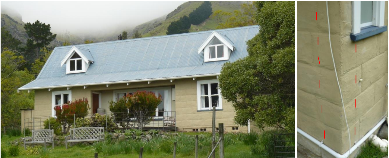
a) Lower storey rammed earth wall panels between reinforced concrete foundations, bond beams, and columns. Rammed earth walls plastered and scribed to appear as blocks. b) Minor wall and plaster cracking at interface to the concrete column.
