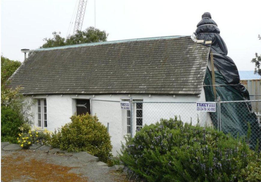
a) Lower parts of walls made of sod, upper walls predominantly cob, cement plaster. Exterior cracking of plaster in a number of places. b) Chimney damage from initial event. Maria Adamski Christchurch City Council
