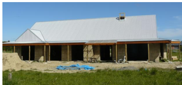
Figure 13: Sandy Knolls Poured Earth House (Building 5). 2010 Vertically reinforced only but no damage evident.
