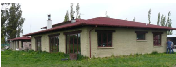
a) 500 m 2 rammed earth house with second level over garage
