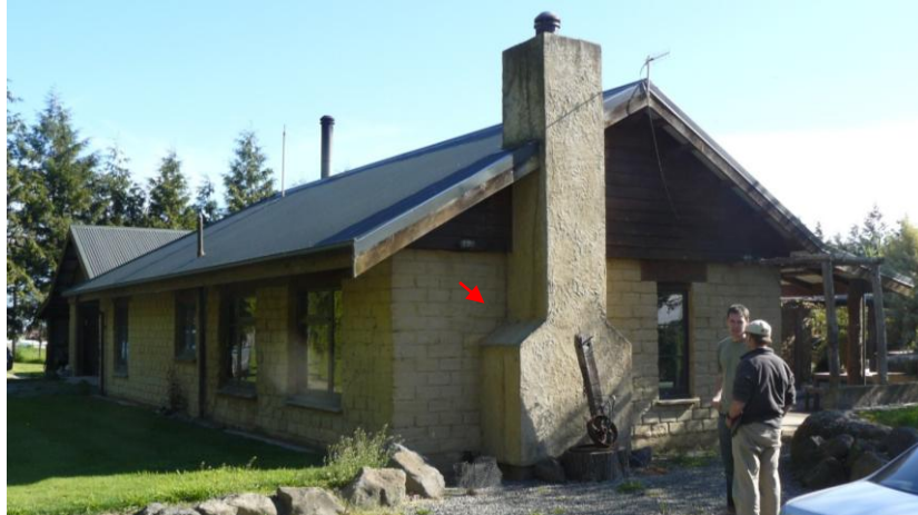
Figure 10: Charing Cross Adobe House (Building 4) 1999. Located between the epicentre and major fault rupture. Reinforcing similar to that specified in the NZ Earth Building Standards. Minor cracking mostly due to differential ground movement.
