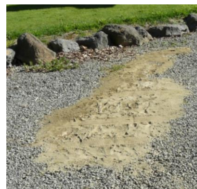
b) Evidence of liquefaction related to differential movement in foundations and cracked paths.
