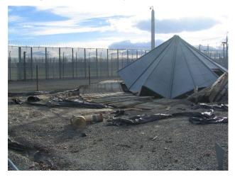
Figure 6: Collapsed timber tank.
