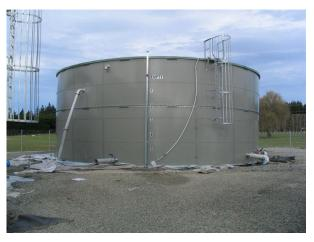
Figure 7: Damaged bolted steel tank.
