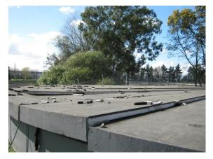
Figure 4: Reservoir roof damaged by convective wave.
