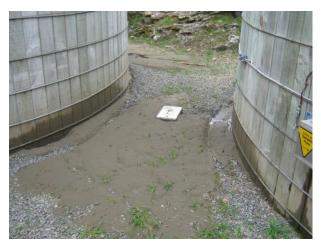
Figure 5: Timber tanks with ruptured liners.
