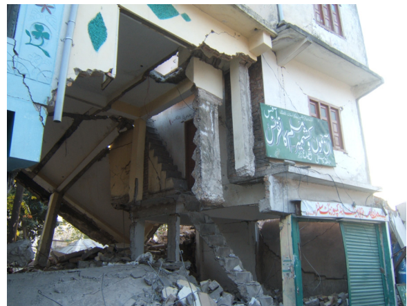
b) Reinforced concrete frame building on top of masonry building.
