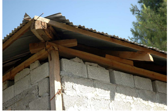
b) A block masonry building with light timber frame constructed after earthquake (note change in walls after earthquake).
