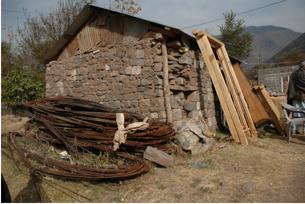
a) A stone masonry building with light timber frame , damaged by earthquake.
