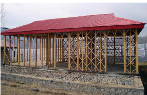
a) A Dhajji under construction.
