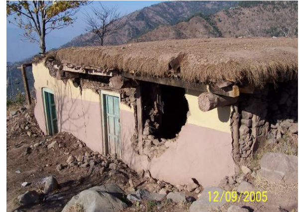
b) A traditional stone masonry building
