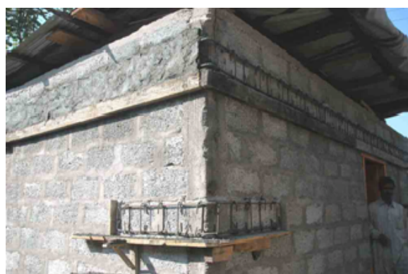
b) Implementing remedial measure for seismic safety.
