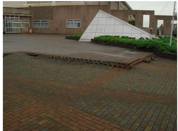
Figure 11: Damage to Kashiwazaki Aquapark. Top photo shows uneven settlements in the perimeter of the building and lateral separation of the walls; bottom photo shows the settlement of the pavement in front of the building.
