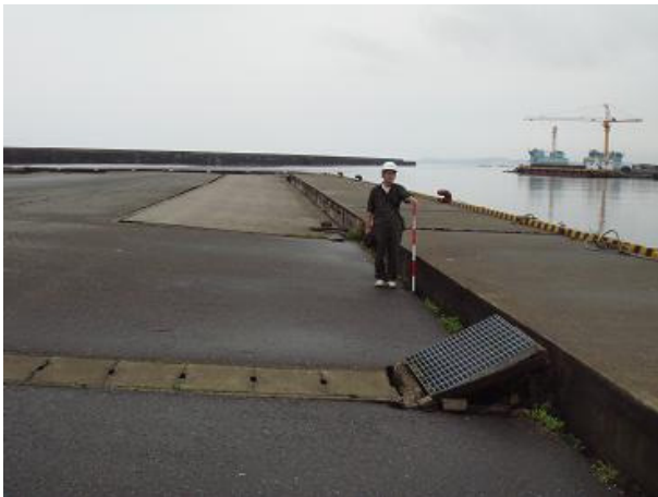
Figure 10: Damage to Kashiwazaki Port. Top photo shows lateral spreading of the quay wall towards the sea while bottom photo shows settlement of the apron.
