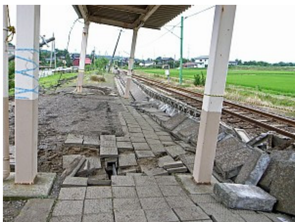
Figure 12: Damage to railway facilities: top photo shows the buckled railway track while the bottom photo shows the damaged platform of Arahama train station.
