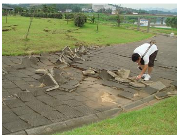
Figure 9: Sand boils and ground fissure observed in Sabaishigawa Memorial Park.
