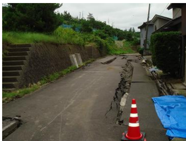
Figure 7: Liquefaction-induced ground deformations in Yamamoto Danchi, Yamamoto town.
